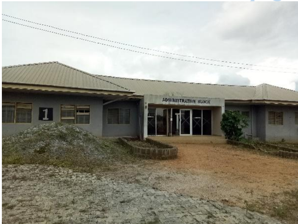
Plate 3.4 : Admin Block, IDC Osogbo
