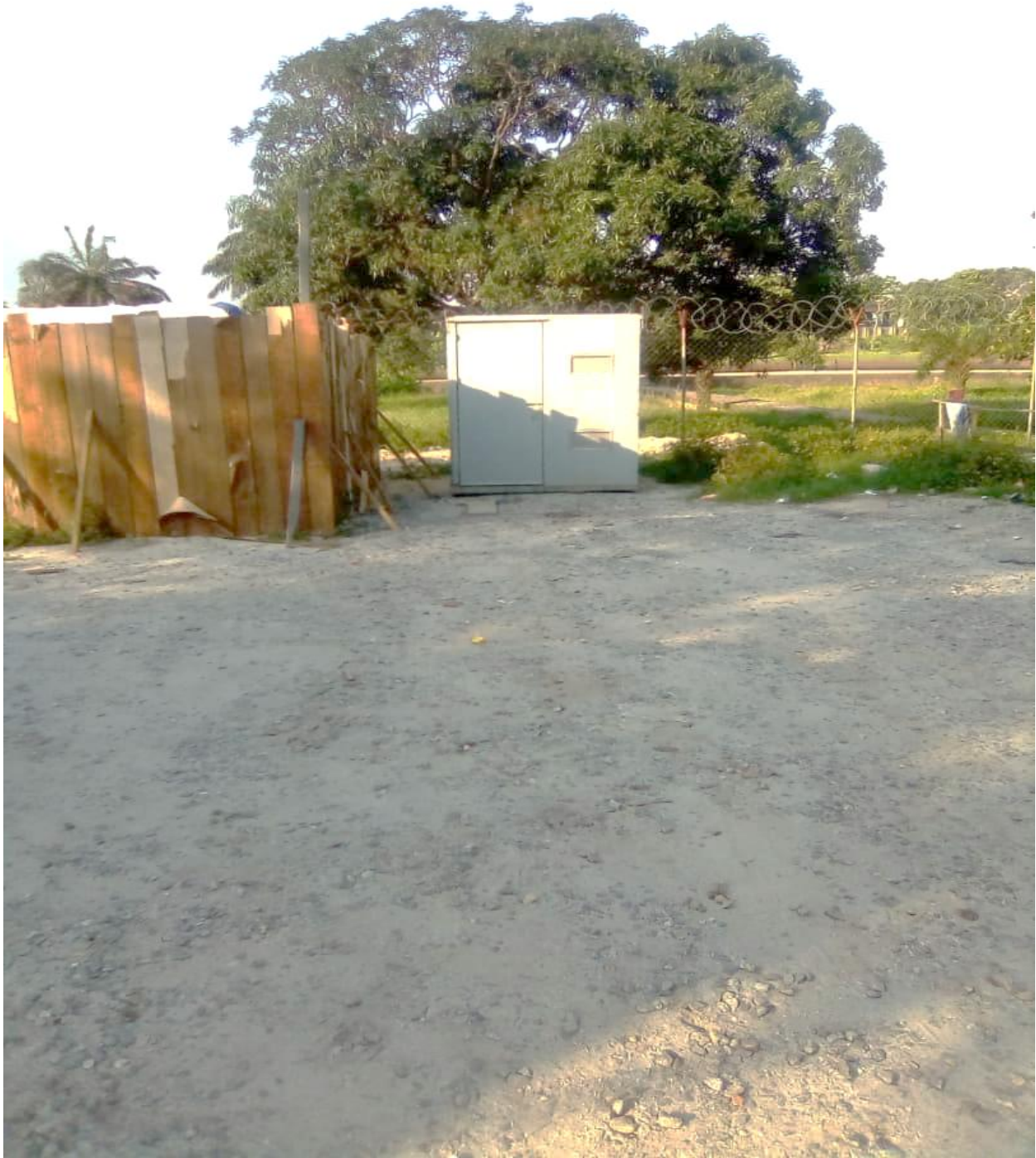
Plate 13: Untarred Park of the Uncompleted New National Arts Theatre, Lagos
