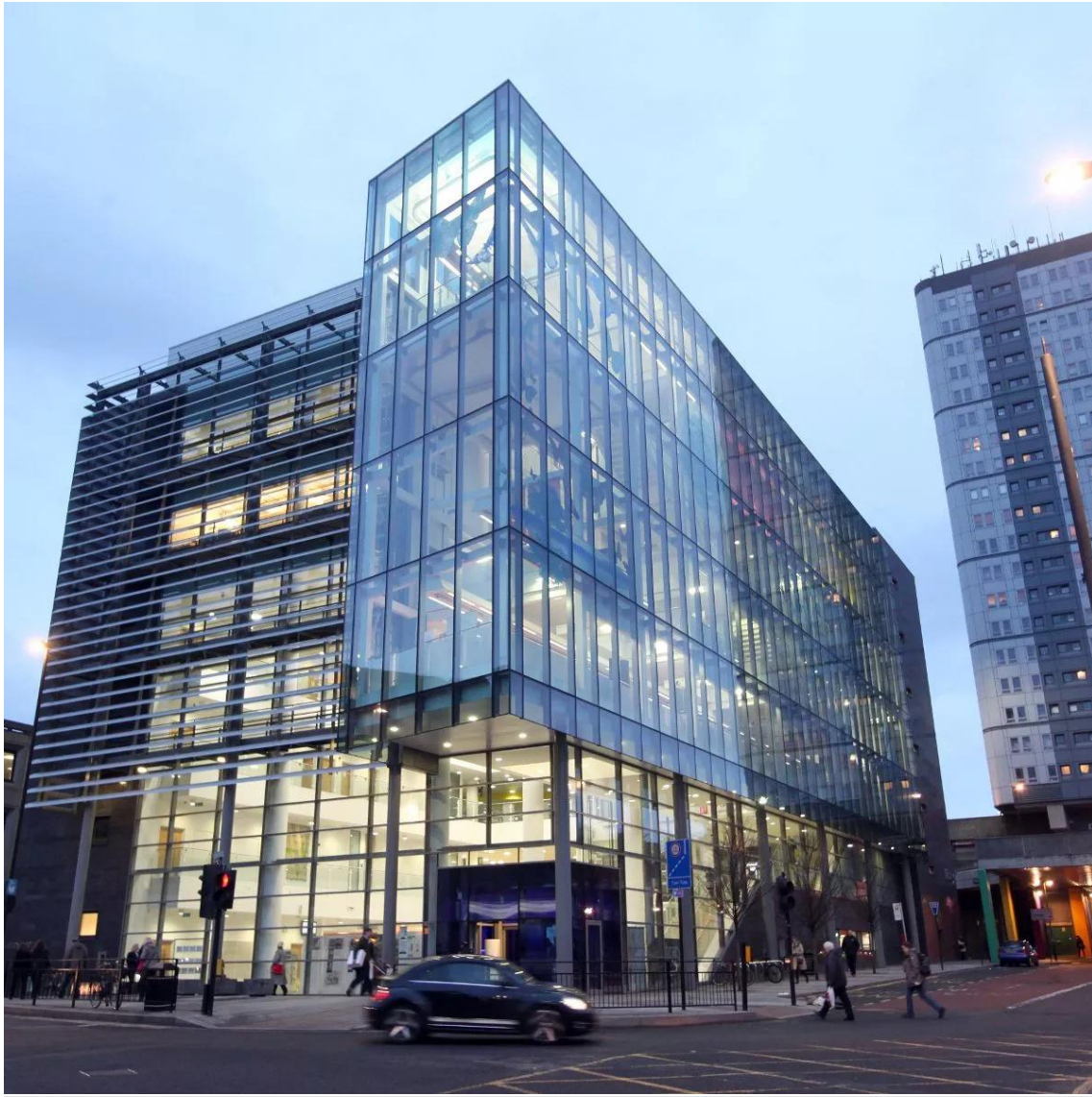
Plate 1.1; Illustrating the exterior view of the Newcastle City Public Library building
