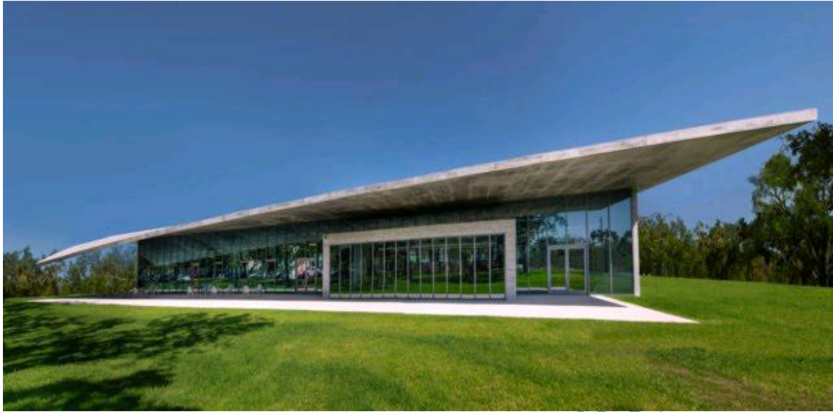
Figure 25; Picture showing wide expanse of fixed glass which gives enough illumination into the building layout of the school of architecture Miami University.
