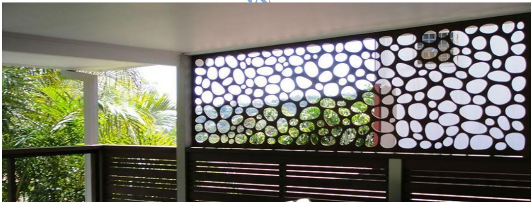
Figure 2.5 Typical Laser Cut Panel System
