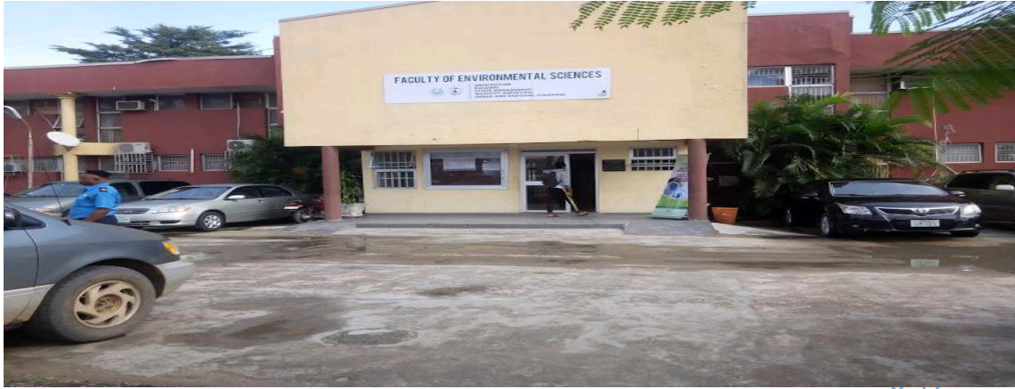
Figure 39; Well celebrated approach view of the faculty with disabled access and adjoining packing lots.
