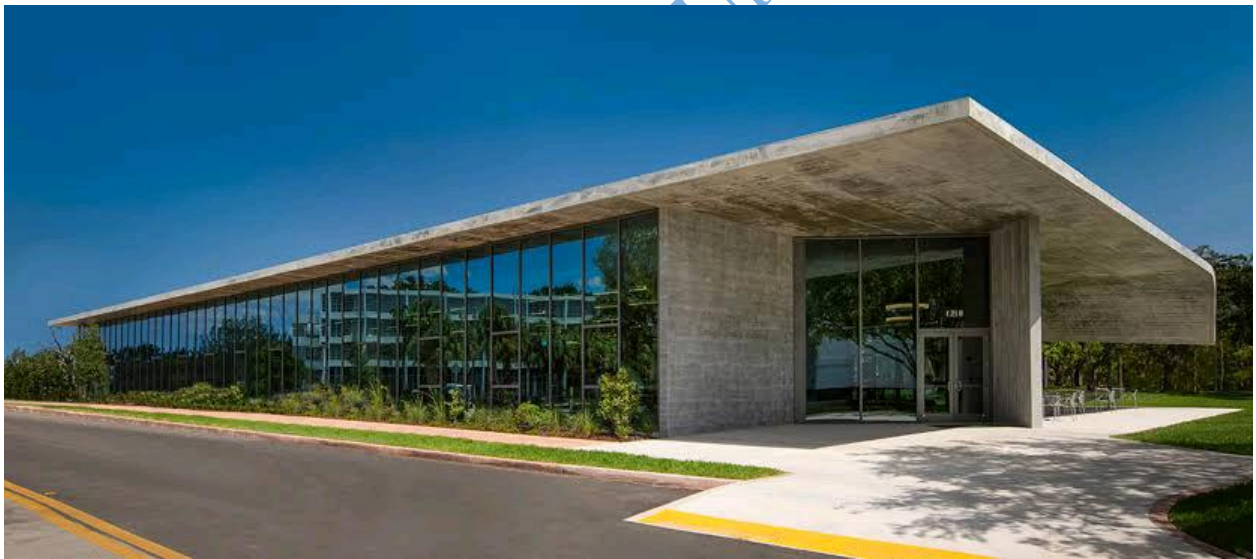
Figure 24; Approach view of the school of architecture with adjoining road
