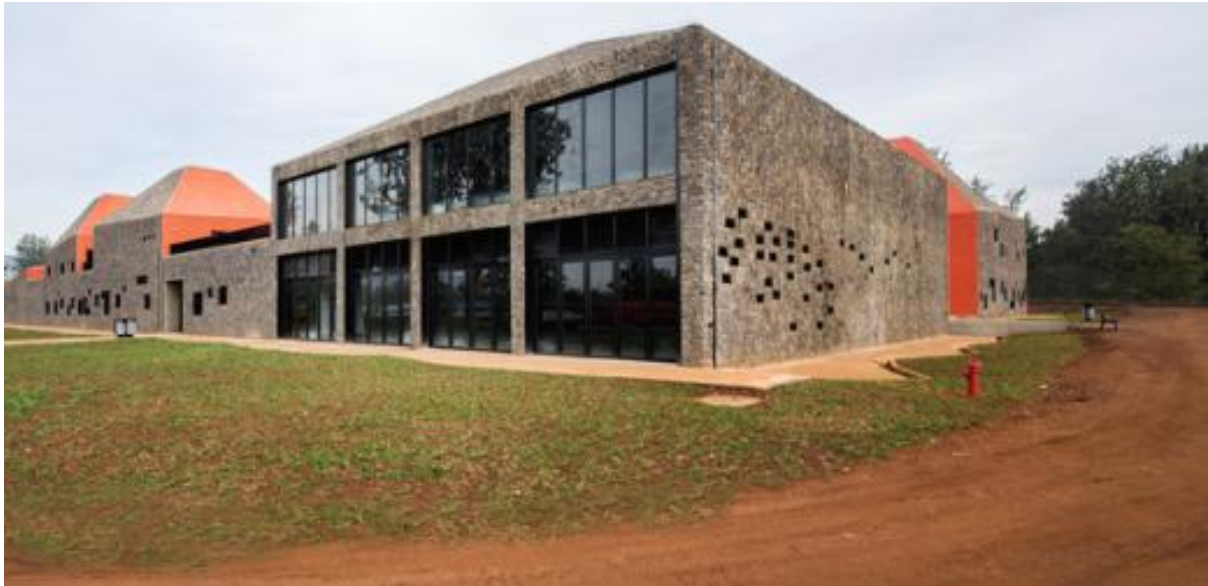
Plate 3.3.3 Case Study 1: Exterior southwest side of the university of kigali, rwandaSource: ArchDaily (2024)
