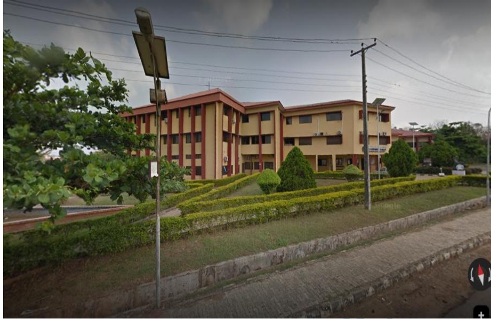
Plate 3.3.15: Exterior of federal university of Technology Akure, (Fieldwork2024)
