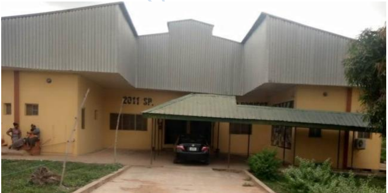
Plate 28: Approach view of Gani Bello Library, Federal College of Education, Abeokuta, Ogun State.
