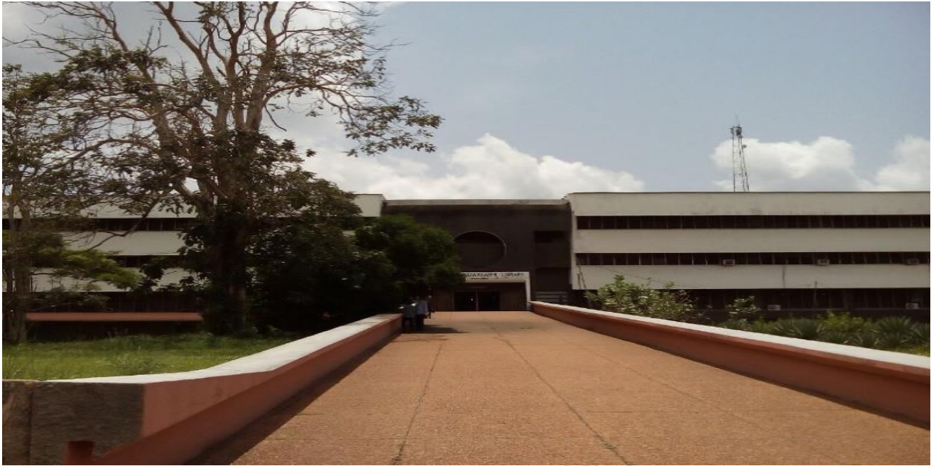
Plate 15: Ramp at the entrance of Hezekiah Oluwasanmi Library, Obafemi Awolowo University, Ile Ife, Osun State.
