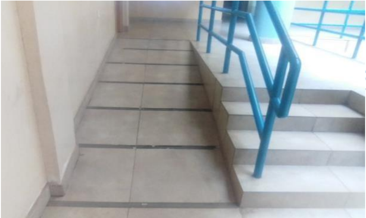
Plate 22: The interior ramp in Timothy Olagbemi Library, Bowen University Iwo, Osun State.
