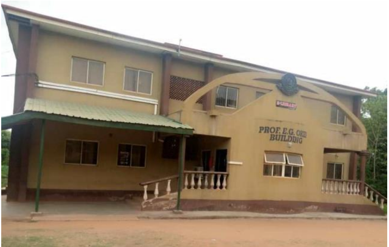
Plate 31: Approach of the E Library, Federal College of Education, Abeokuta, Ogun State.
