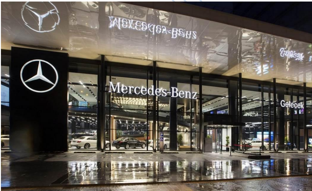
Plate 13: Façade of Mercedes-Benz Vadi Park Showroom Source: ArchDaily App, 2022.
