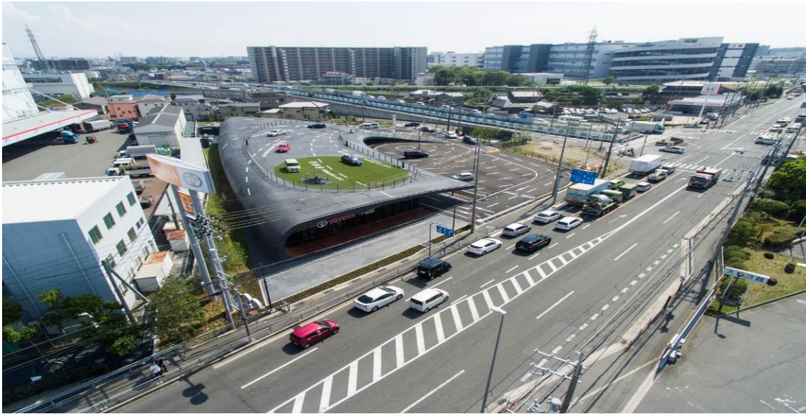
Plate 17: Façade of the elevated outdoor display ramp platform of Toyota Corolla Shinosaka Meishin Ibaraki Showroom
