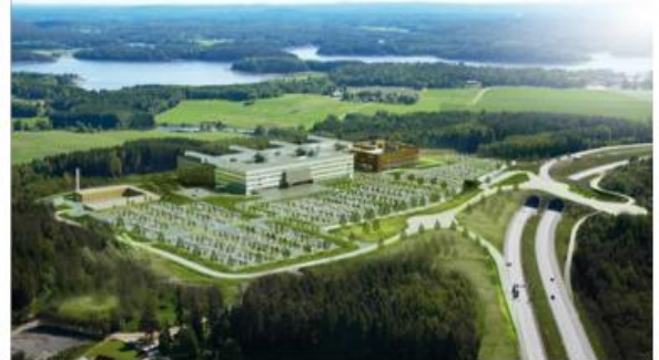
New Østfold Hospital, Sarpsborg
