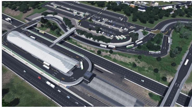
Figure 2.9: Road – Road Interchange Source: ( www.reddit.com ).
