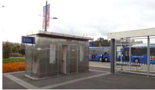
Figure 2.28: Toilet Facilities for customer's comfort. Source: ( www.at.govt.ng ).
