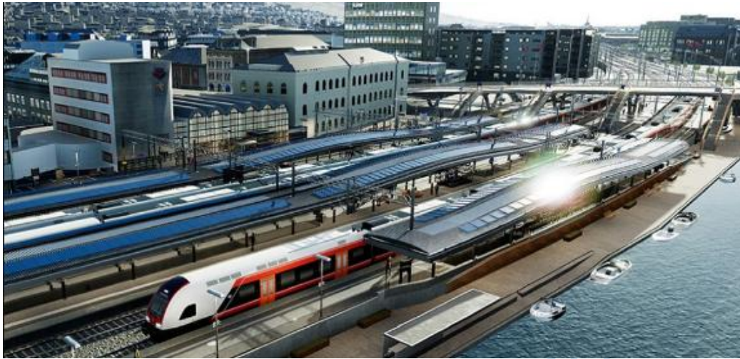
Figure 2.15: Interchange located at considerable distance to one another. Source: ( www.dsl-au.com ).
