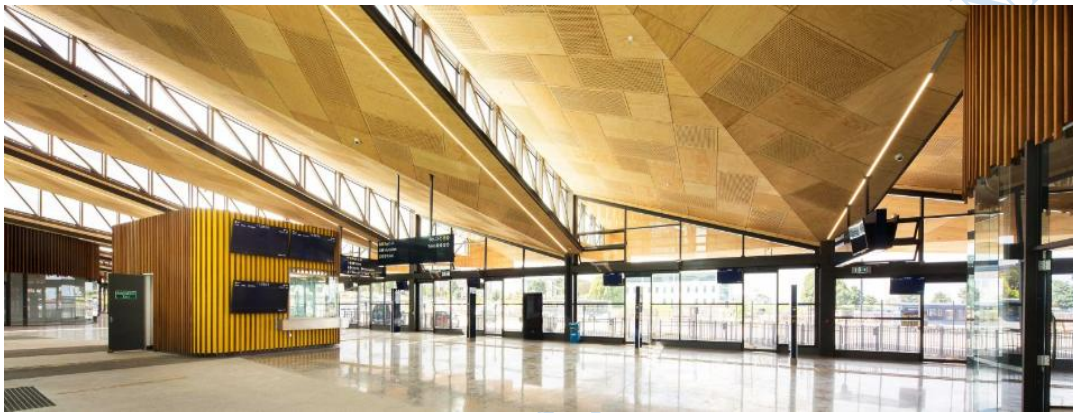
Figure 3.36: Clearstory glazing for natural lighting and fresh air Source: www.greaterauckland.org.nz
