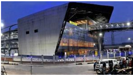
Figure 3.21: Exterior view of the interchange Source: www.autoreportng.com .
