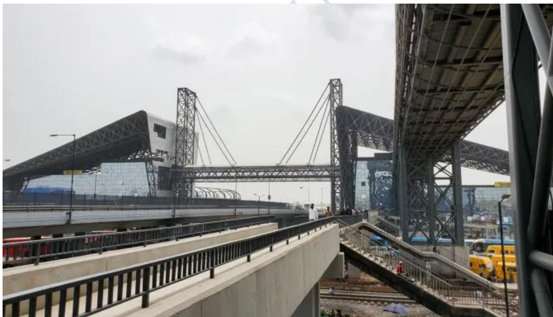
Figure 3.17: Skywalk bridge at Oshodi Interchange
