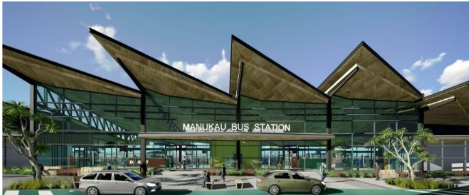
Figure 3.34: Kite like roof structure of Manukau Bus Interchange
