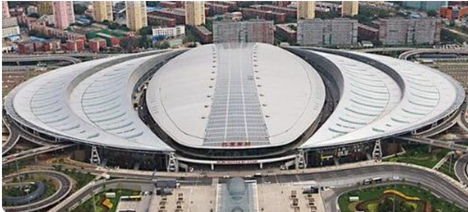
Figure 3.24: Aerial view of Metro Station, Beijing Source: www.pinterest.com .
