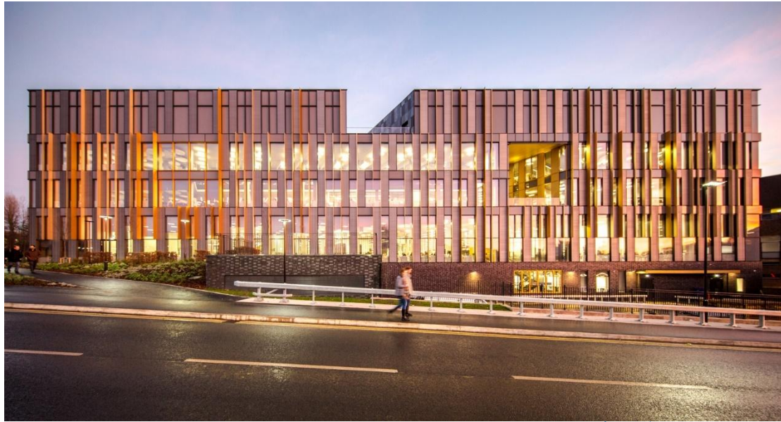
Figure 3.14: Approach view of University of Birmingham's Library
