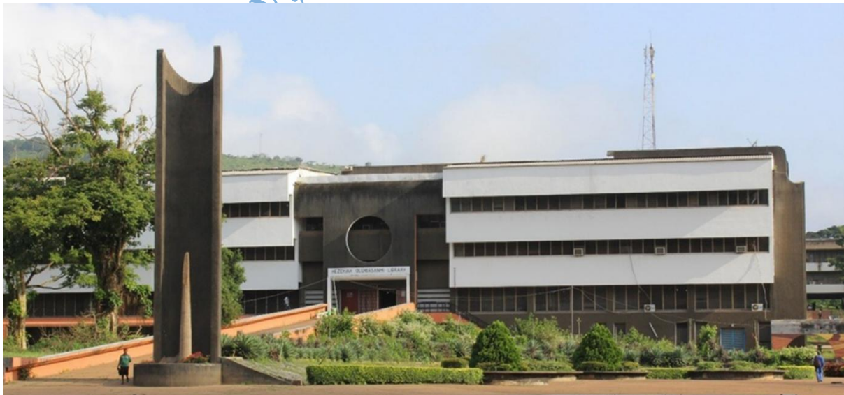
Figure 3.32: Approach view of Obafemi Awolowo University Source: (Researchers Field Work)
