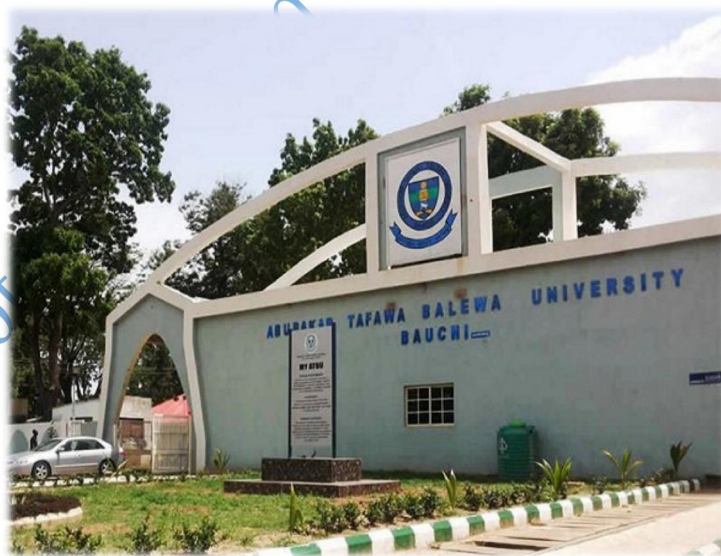
Figure 3.37: Entrance Gate of Abubakar Tafawa Balewa University Library
