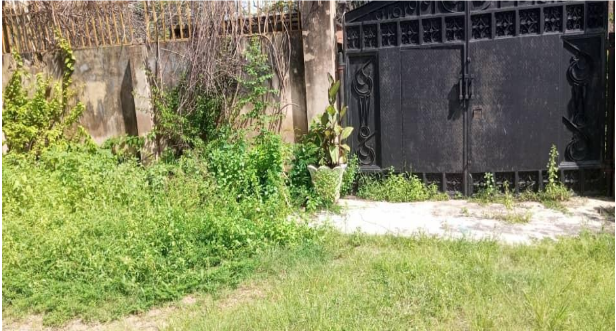
Plate 4.25: Abandoned Residential Buildings at Ibara Housing Estate, Abeokuta
