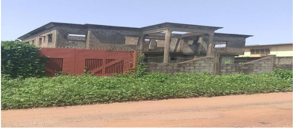
Plate 4.9: Abandoned Residential Buildings at Obasanjo Hilltop Housing Estate, Abeokuta.
