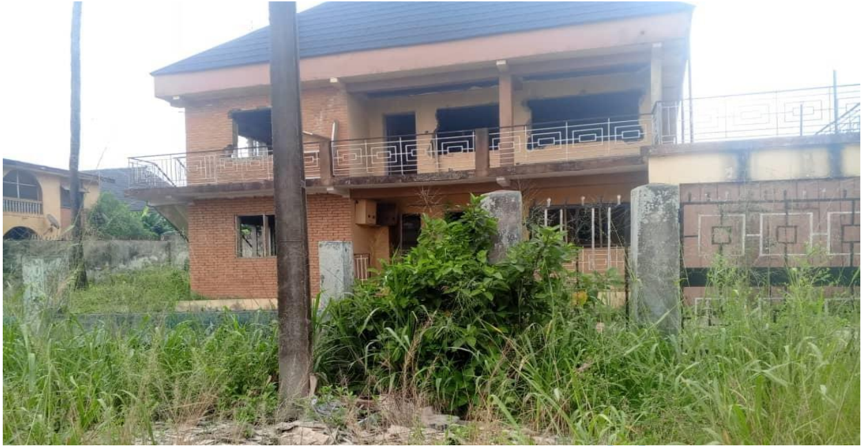
Plate 4.21: Abandoned Residential Buildings along at Asero Housing Estate, Abeokuta.
