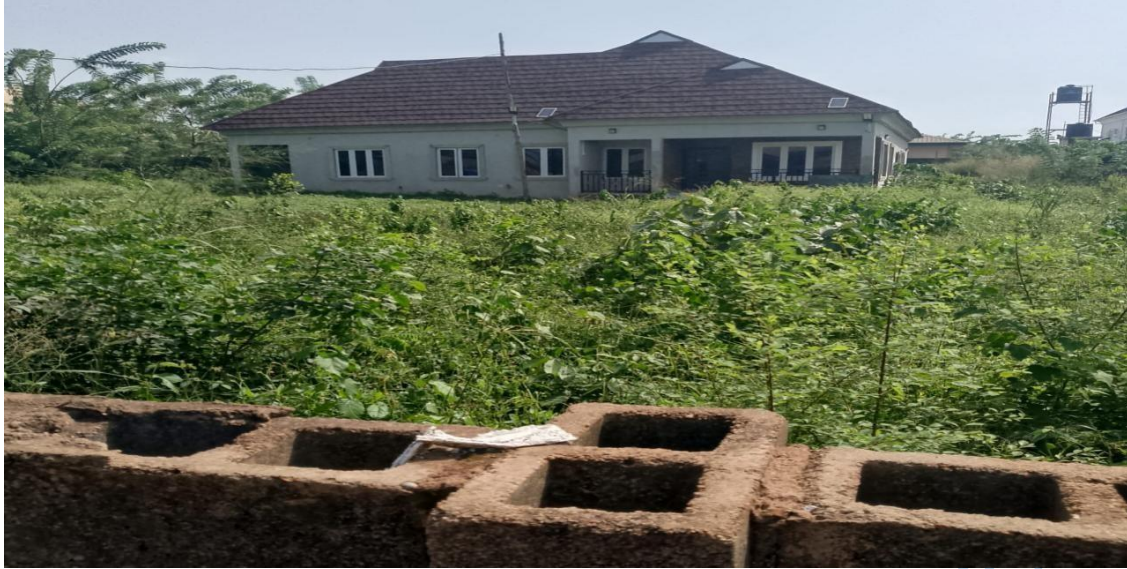
Plate 4.3: Abandoned Residential Buildings at Laderin Housing Estate, Abeokuta
