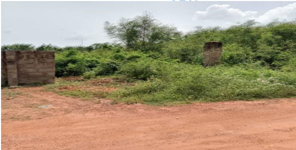
Plate 4.16: Abandoned Residential Buildings at Obasanjo Hilltop Housing Estate, Abeokuta. Source: Field Survey, October, 2024
