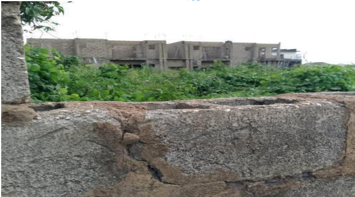
Plate 4.10: Abandoned Residential Buildings at Obasanjo Hilltop Housing Estate, Abeokuta Ogun State.
