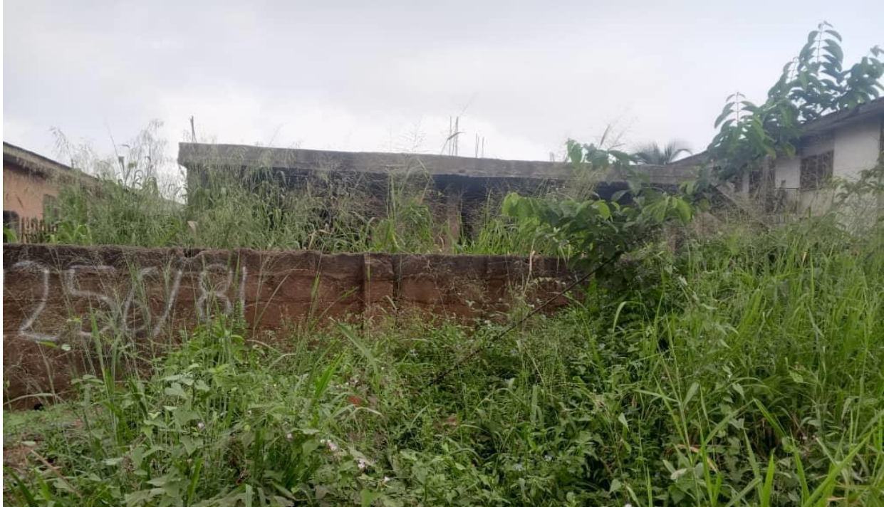
Plate 4.19: Abandoned Residential Buildings along at Asero Housing Estate, Abeokuta.
