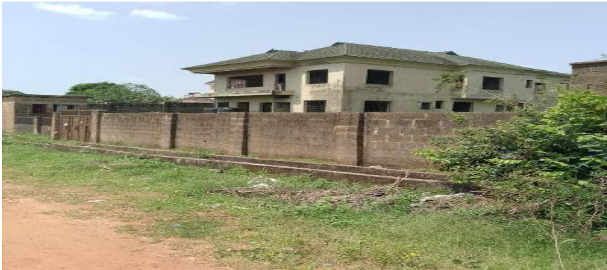
Plate 4.13: Abandoned Residential Buildings at Obasanjo Hilltop Housing Estate, Abeokuta Ogun State.
