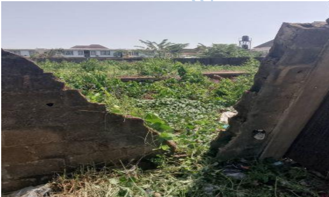
Plate 4.8: Abandoned Residential Buildings at Obasanjo Hilltop Housing Estate, Abeokuta
