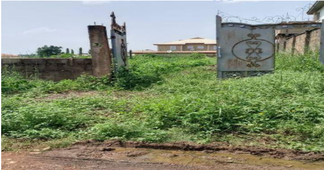
Plate 4.6: Abandoned Residential Buildings at Laderin Housing Estate, Abeokuta Source: Field Survey, October, 2024
