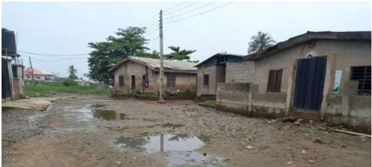
Figure 4.19: Buildings Features in the study area Source: Researcher's Field Survey, (2023)
