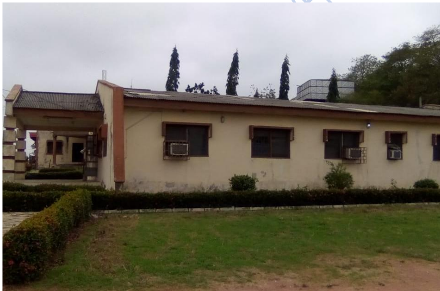
Plate 3: Showing the Side view of the Faculty building, showing openings, vegetation and outdoor units of the mechanical cooling device
