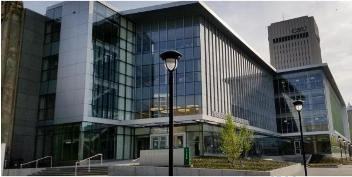
Plate 31: Showing the approach view of Washkewcz College of Engineering, Cleveland State University
