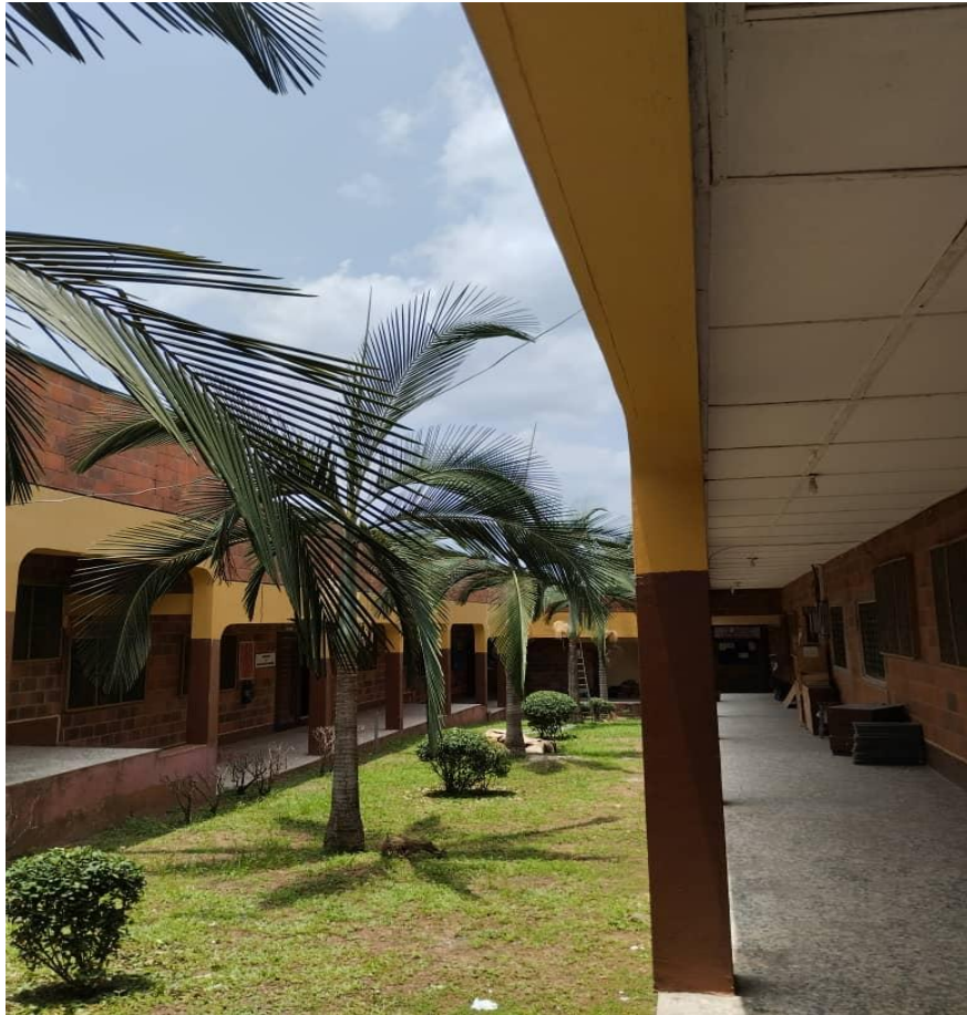
Plate 14: View showing the court yard of the Administrative office block, College of Engineering, Bells University of Technology, Ota, Ogun State.
