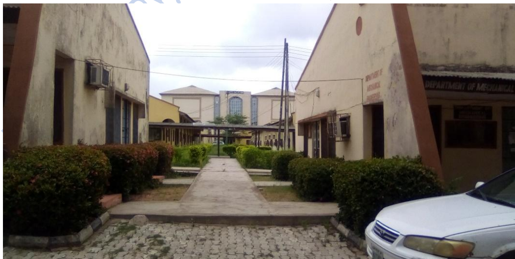
Plate 6: view showing the Faculty of Engineering and Technology, lecture hall known as the High rise building along the departmental blocks, Ladoko Akintola University of Technology, Ogbomoso, Oyo State. Source: Researcher's Field Work, 2022.
