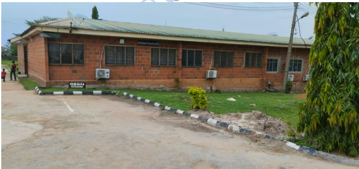
Plate 13: View showing the Administration block of the college of engineering, Bells University of Technology Ota, Ogun State.
