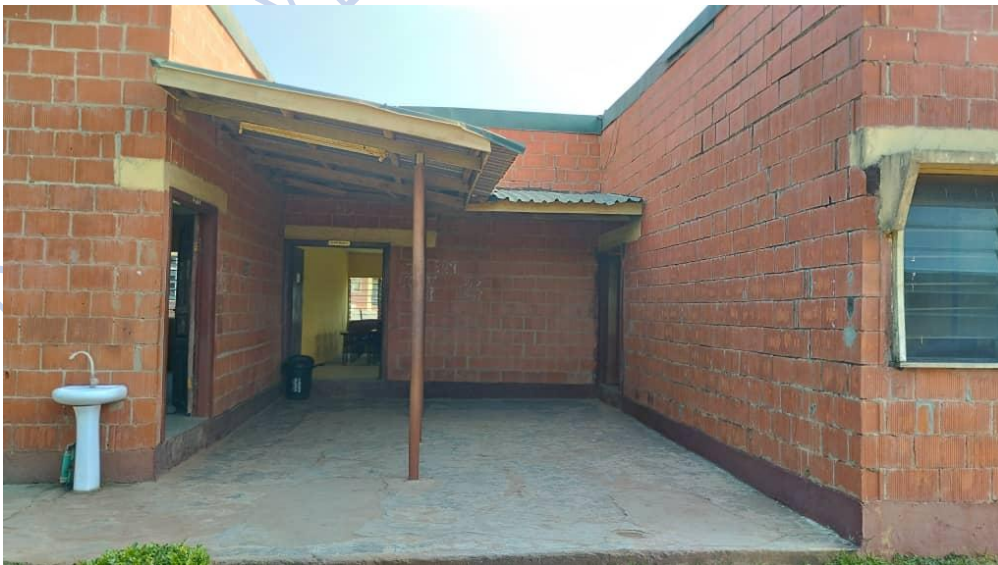
Plate 20: Showing the approach view of the lecture room, college of engineering, Bells University of Technology Ota, Ogun State.
