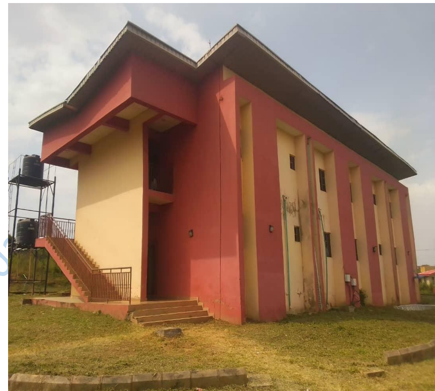
South-East View of El-Salem Hall, Abiola Ajimobi Technical University, Ibadan
