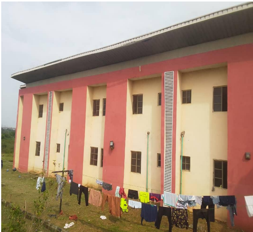
North-West View of El-Salem Hall, Abiola Ajimobi Technical University, Ibadan.
