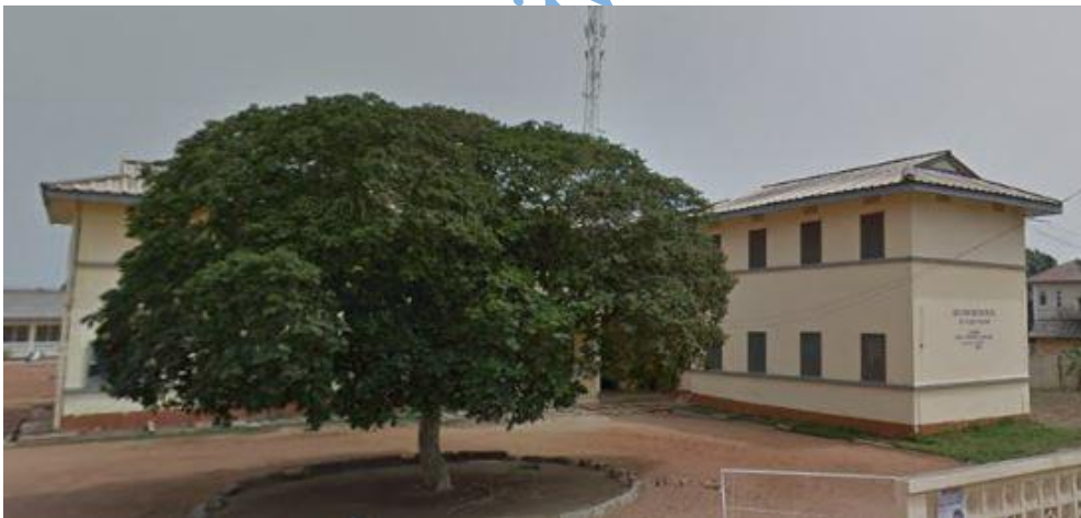
Figure 3.15: Building Exterior. Source: google search
