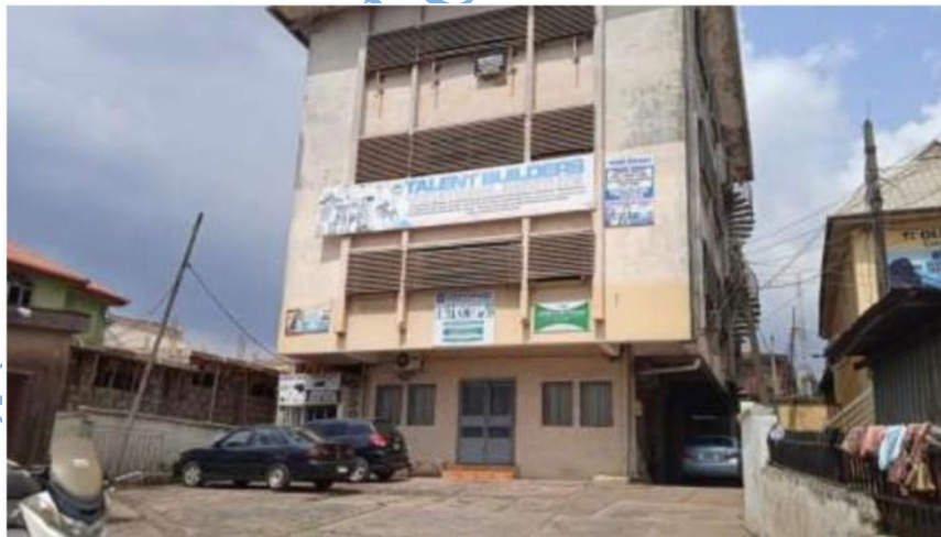
Figure 3.6: Exterior of building showing poor landscaping.
