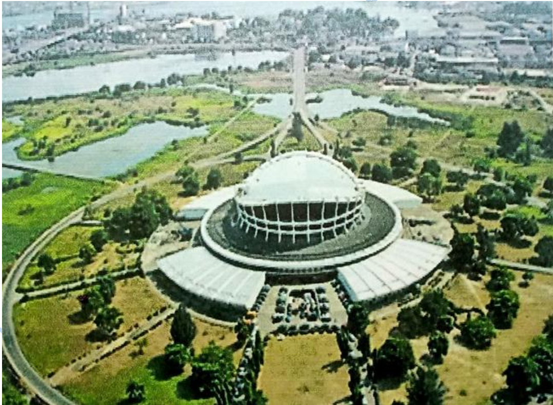
Plate 5: Aerial View, National Art Theatre, Lagos Source: Author's Survey, 2024
