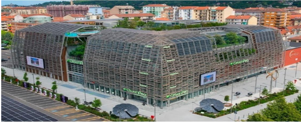
Figure 3.29: The 3-D view showing the building external envelope of wooden sunshade slat supported by steel ribs to form a technical treillage acting as a filter between inside and outside.
