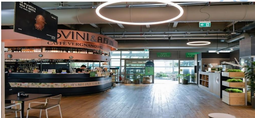
Figure 3.30: The interior view showing the parquet made of wood and suspended ceiling with conducted services connections and LED lamps.
