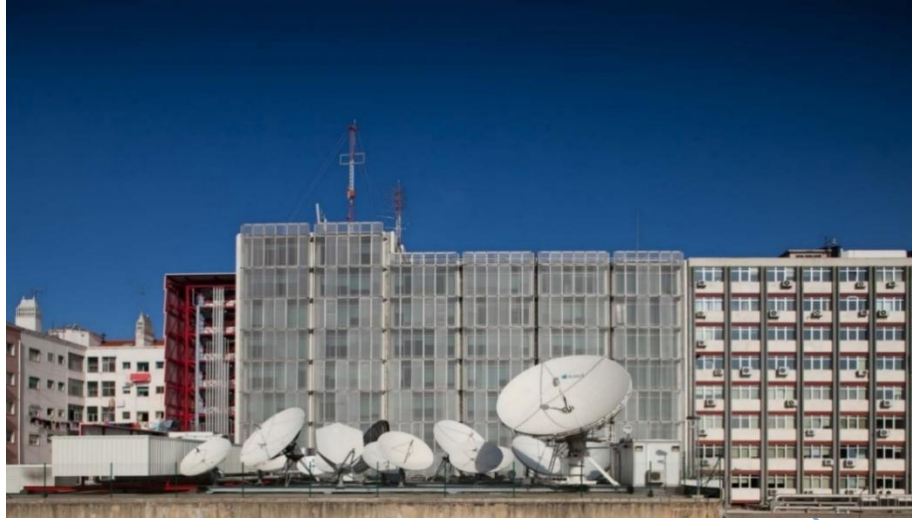
Figure 3.11 : Exterior view of Telecom Office Building, Portugal Source- (Francisco Nogueira)
