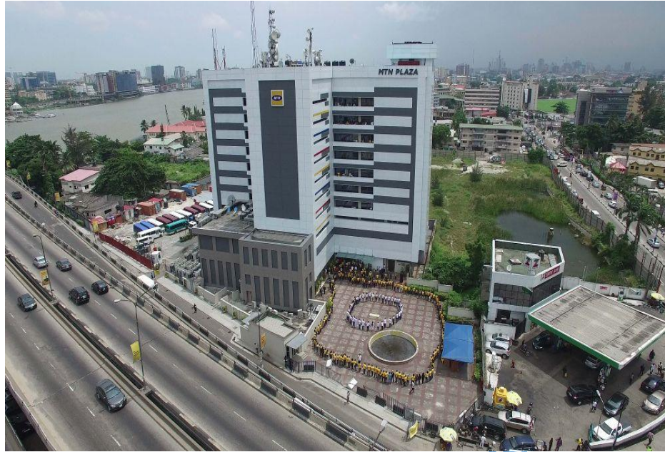
Figure 3.17 : Existing Retrofitted MTN PLAZA Office Source- (Adeniyi Coker Consultants Limited (ACCL))
