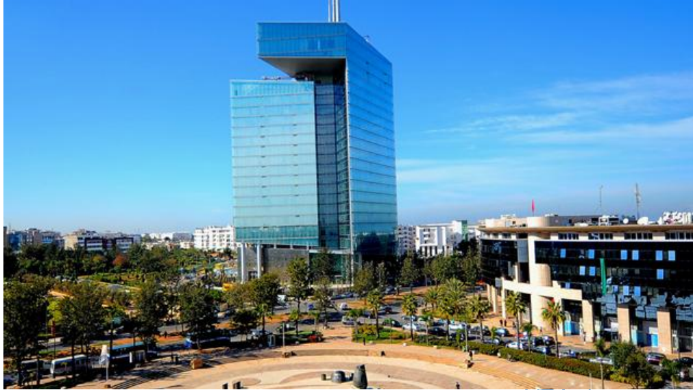
Figure 3.6 : 3d view of the Maroc Telecom Building Source- (Takuji S)
