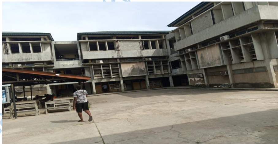
Plate 3.16: Courtyard of Faculty of Engineering, University of Lagos
