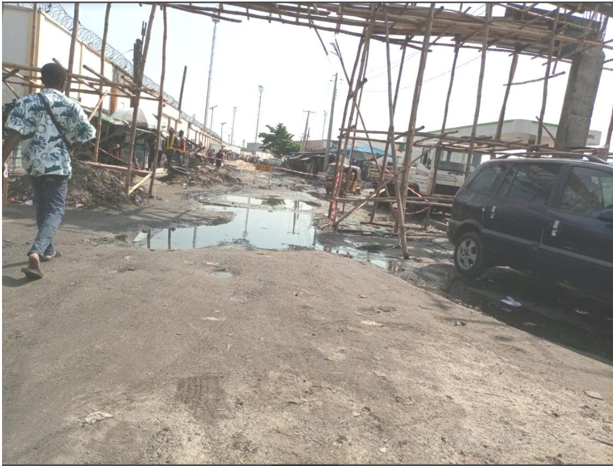
Side view and frontage of a government facilities in two of the slum settlements of Lagos State
