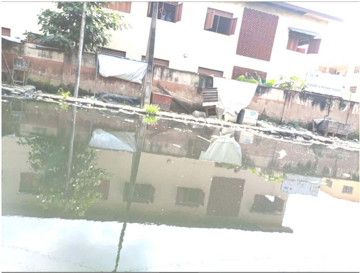
A back view of a government facility in the slum area in the Lagos State metropolis
