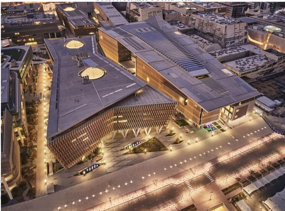
Plate 3.9 Exterior View of the College of Life Sciences Source: Author's Fieldwork
