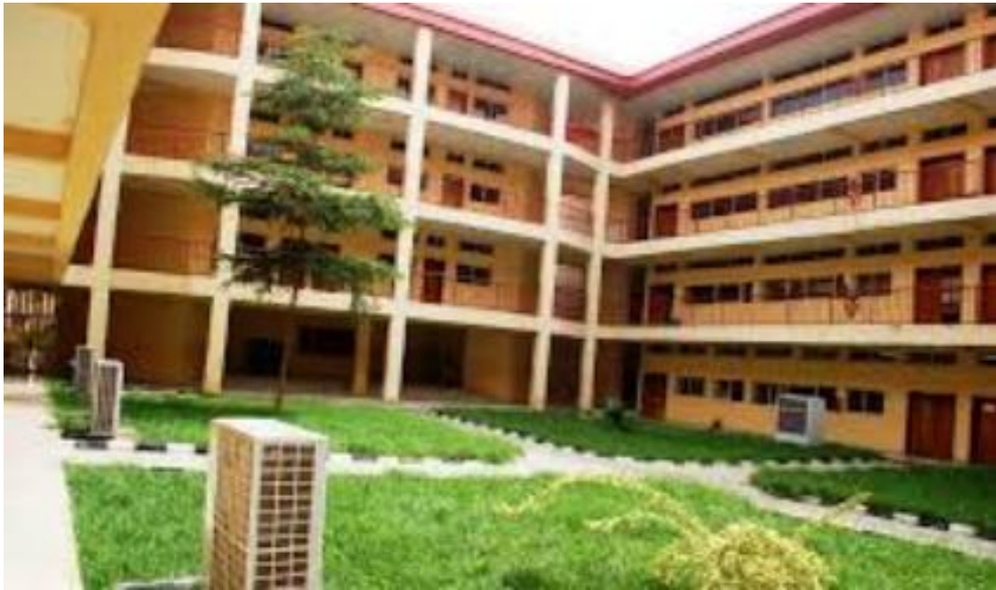
Plate 3.4: Showing Courtyard of the Faculty Building Source: Author's Survey
