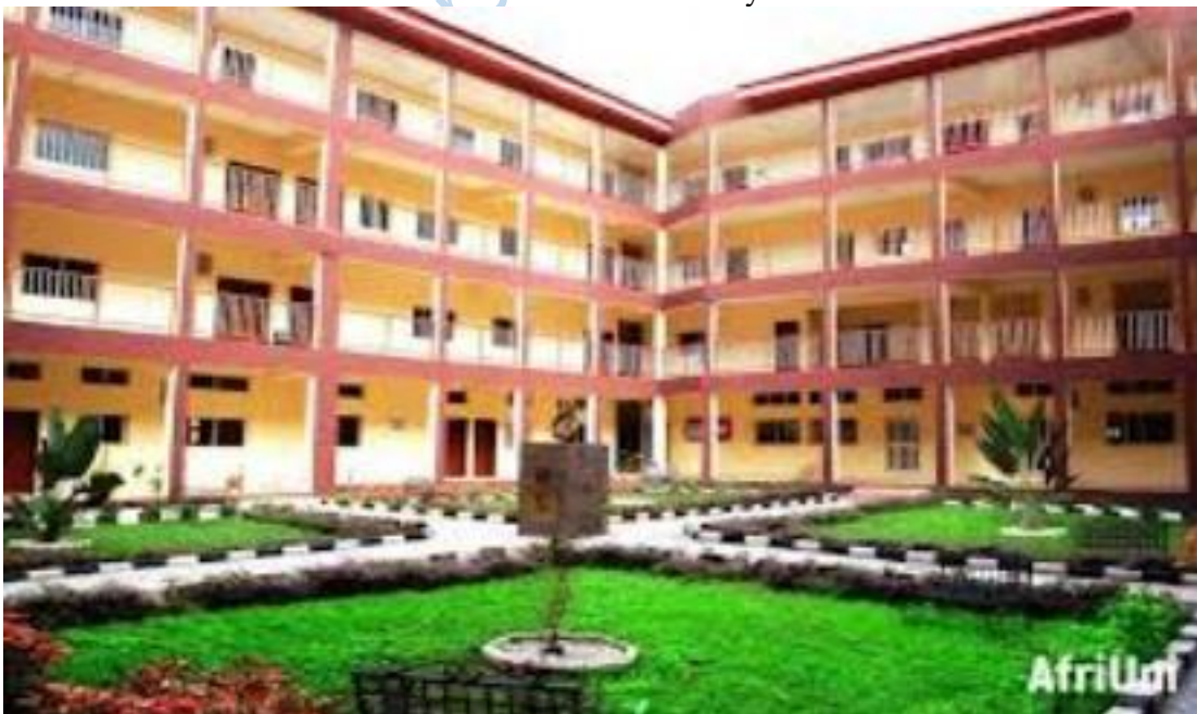
Plate 3.3: Showing Courtyard of the Faculty Building Source: Author's Survey
