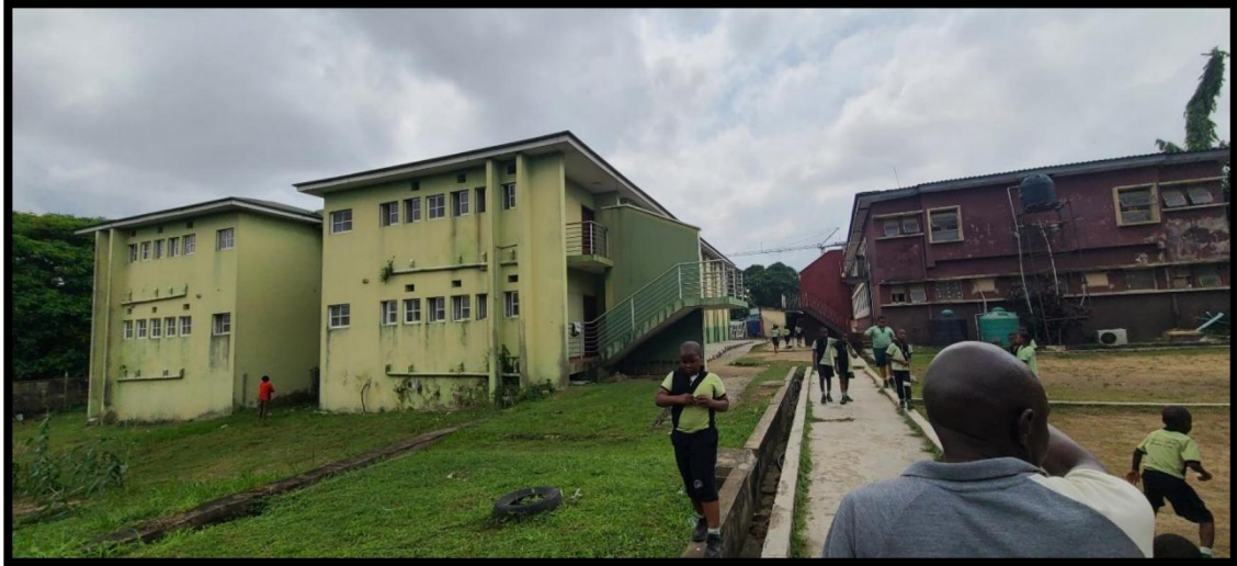
Plate 3. 4 : Picture Showing the Exterior of University of Lagos Staff School.
