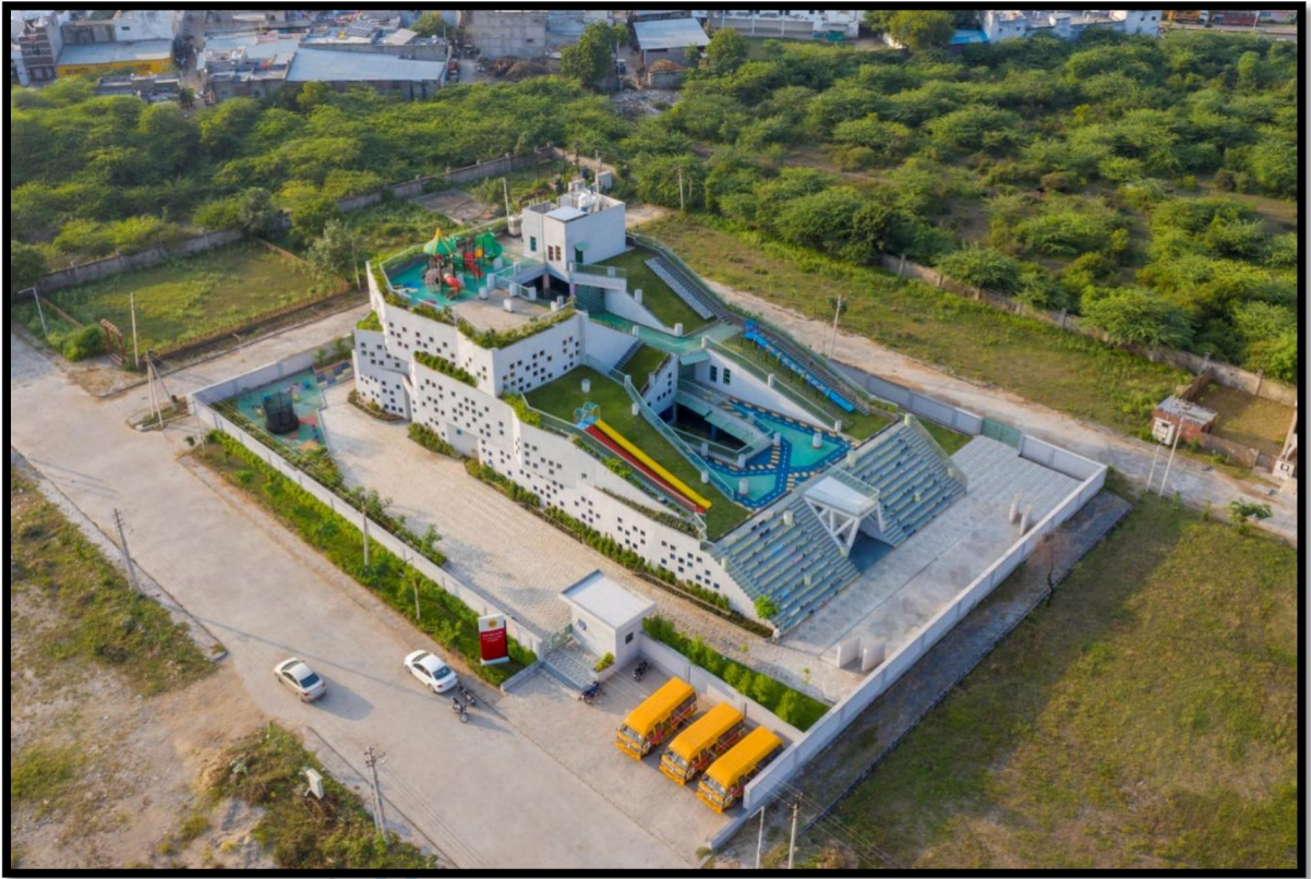
Fig 3.11: Picture Showing the Exterior of Sangam Elementary School.
