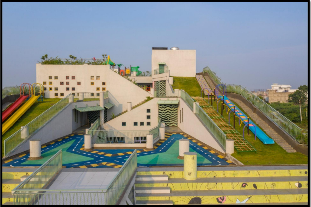
Fig 3.16: Picture Showing the Exterior of Sangam Elementary School.
