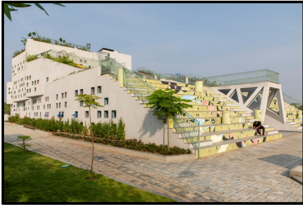
Fig 3.10: Picture Showing the Exterior of Sangam Elementary School.
