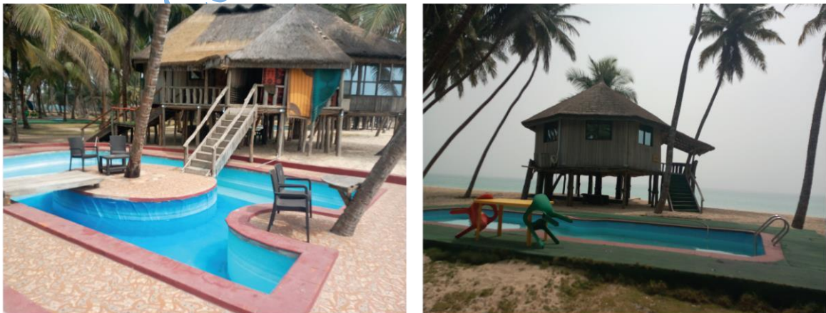
Fig 3.18 The exterior views of the lodging facility called the Putt-Putt
