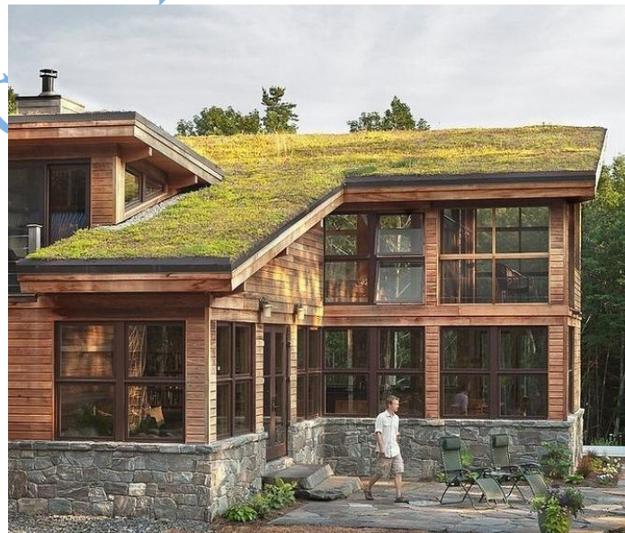
Showing natural materials used in a building
