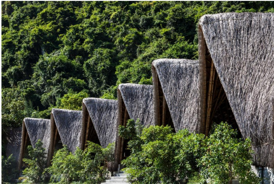
Fig 3.38 Image showing bamboo frame of the accommodation
