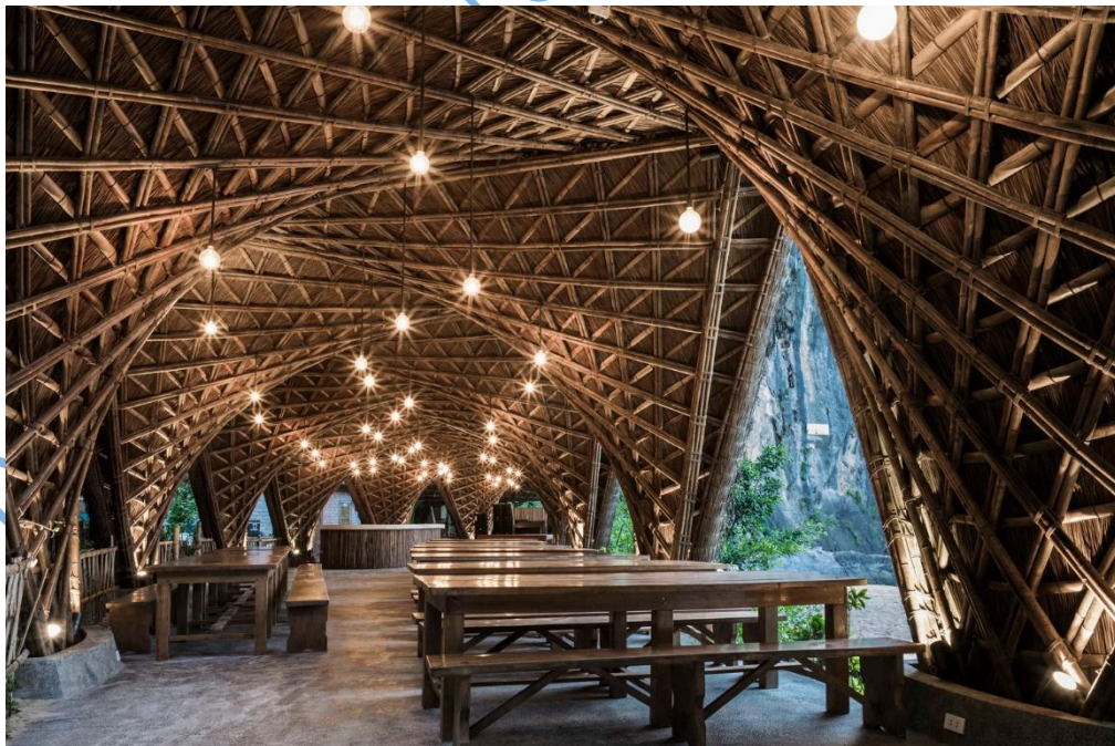
Fig 3.37 Images showing Bamboo shell roof Source: archdaily
