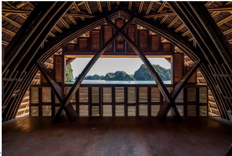
Fig 3.40 showing the room
