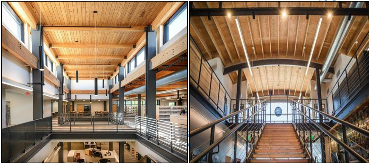
Figure 3.29: Timber and Steel Construction of Rancho Cielo Vocational Center Source: Fieldwork, 2023
