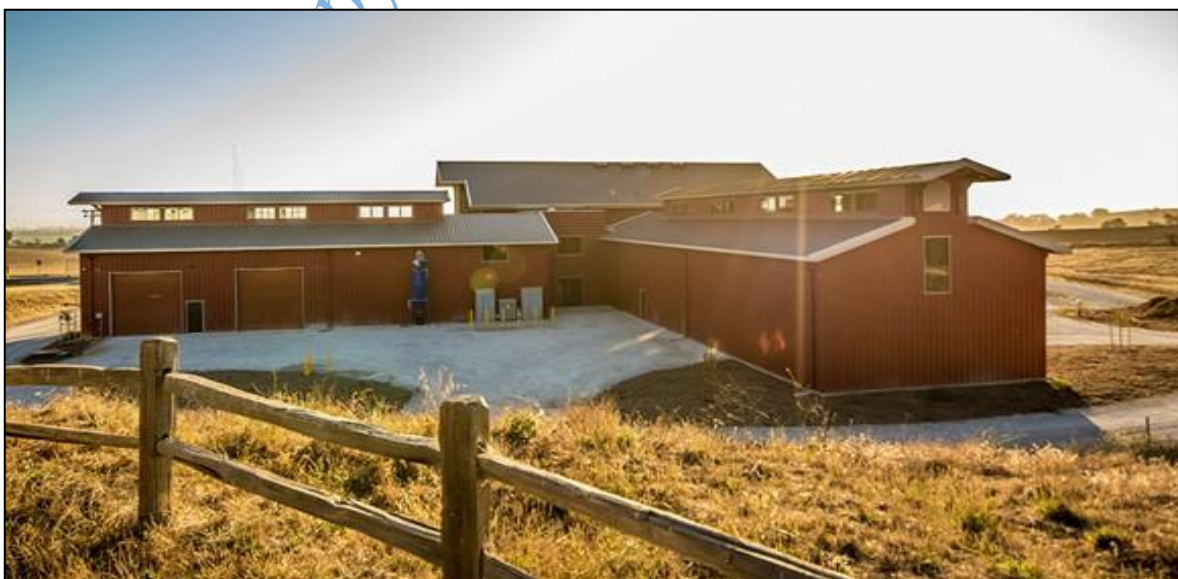
Figure 3.30: Roof Lighting of Rancho Cielo Vocational Center
