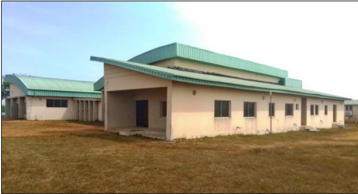
Figure 3.19: Landmark Water Production Factory Source: Fieldwork, 2023
