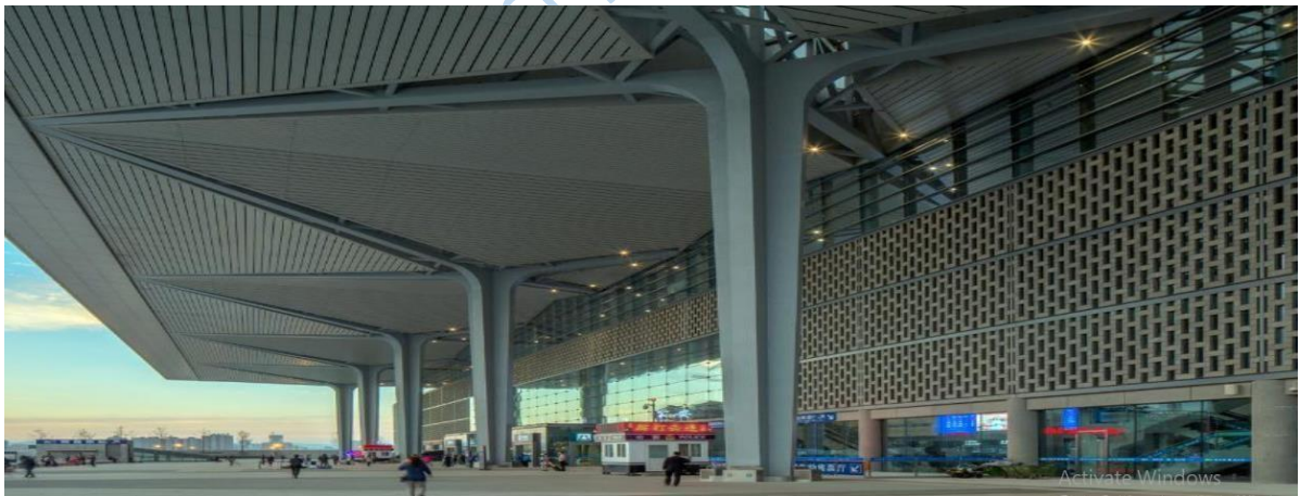
Figure 3.2: Façade of the Taiyuan South Railway Station, China (Source: Archdaily.com, 2024)
