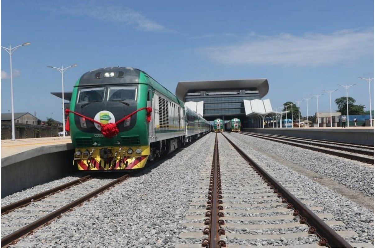
Plate 3.2: Rail Track of the Mobola Johnson Train Station Lagos (Source: Researcher's Field Work, 2024)
