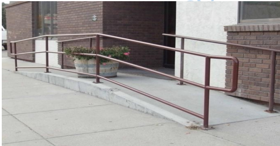
Plate 2.5: Ramp as Accessible Component.
