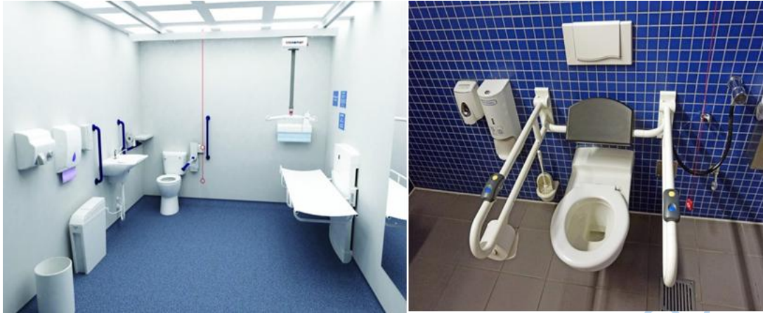
Plate 2.7: Accessible Toilets Grab Bars for Support
