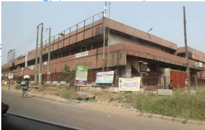
Plate 4.2: Image showing side view of abandoned Agbowo Mall Source: Researcher's Archive, 2023
