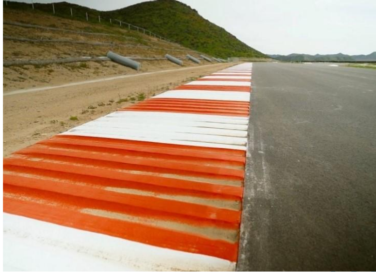
Figure 3.16: Safety Barrier of K1 Speed (Outdoor Track)
