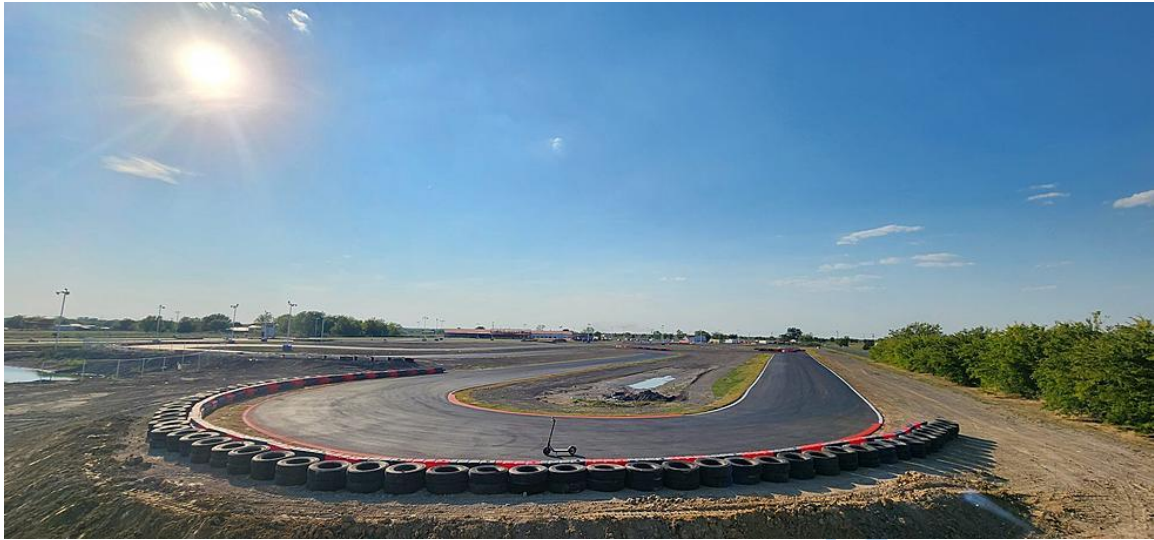
Figure 3.4: Safety Barrier of Dallas Karting Complex
