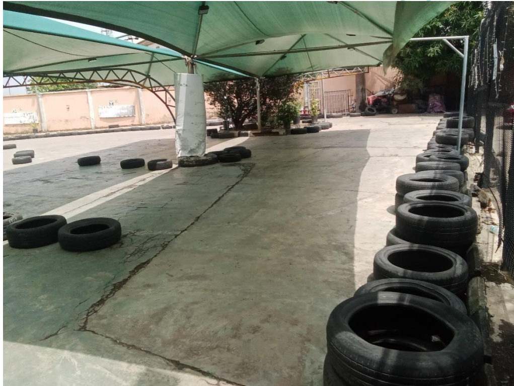
Plate 3.3: Picture Showing the Safety Barrier at Go Kart Arena (Pentorise)
