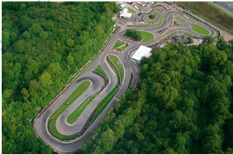
Figure 3.18: Aerial View of Buckmore Park Kart Circuit
