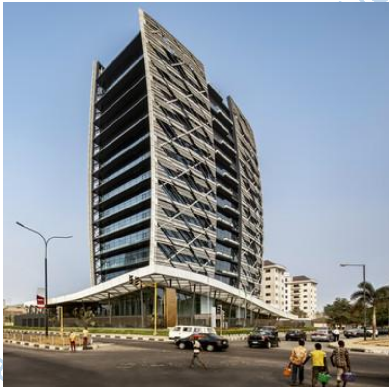
Plate 3.14: Street views of Kingsway Tower
