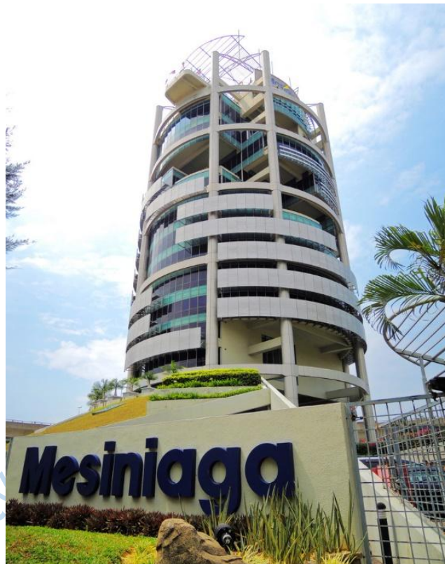
Plate 3.11: Exterior of Mesiniaga Tower
