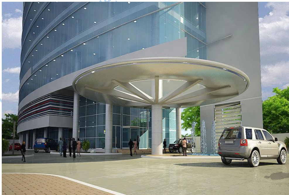
Plate 3.6: Nestoil tower entrance
