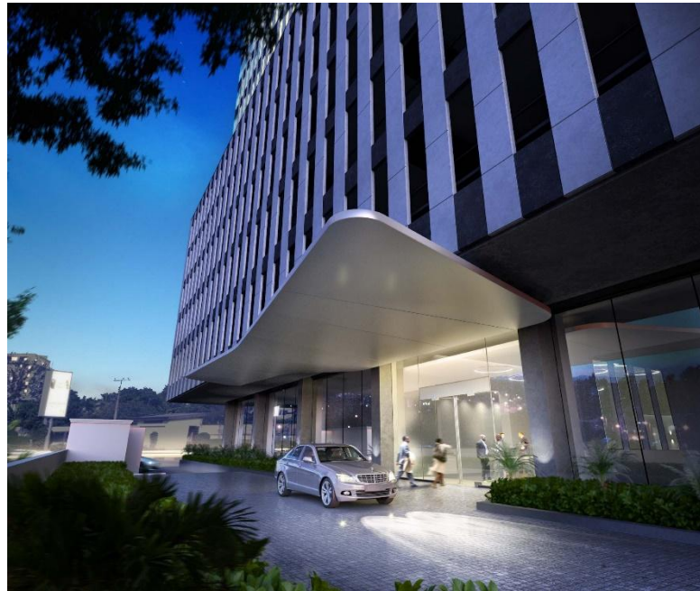
Figure 3.1 : Exterior View of the office Building
