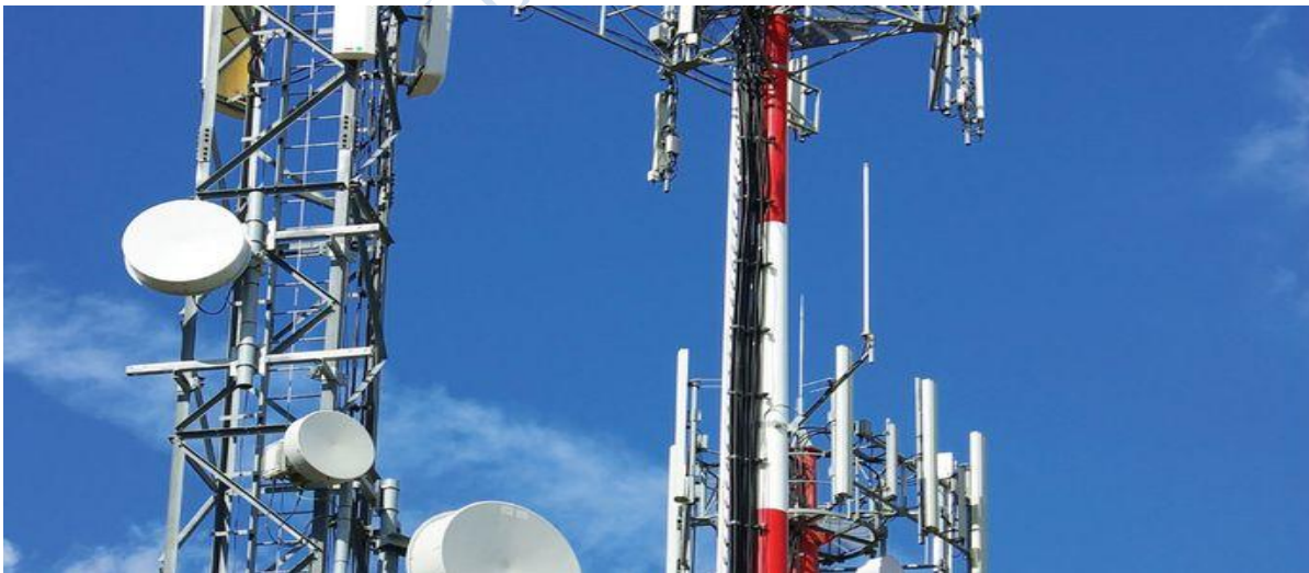
Cell phone tower (right) and combination cell phone and microwave tower (left).
