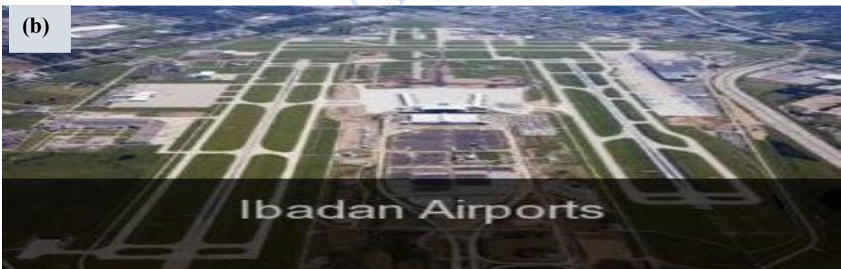
Figure 1.4: (a) Typical Airport Components and Terminal Configurations ; (b) Aerial Photograph of Ibadan Airport 14 .
