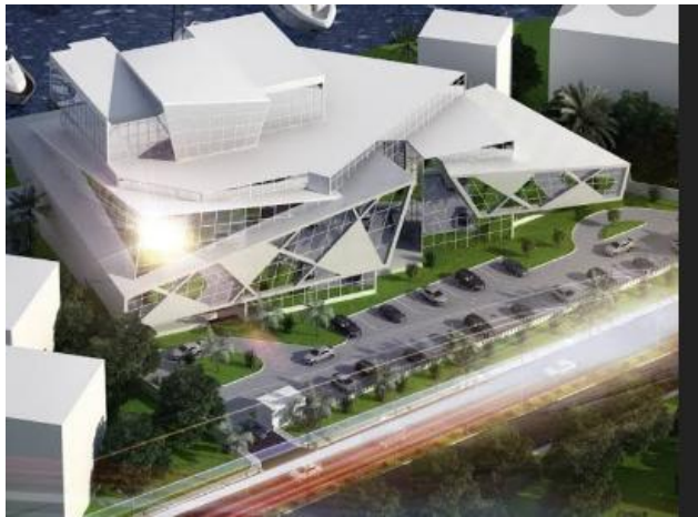
Plate 3.30: Showing Aerial view of Abuja film City Source: Google search
