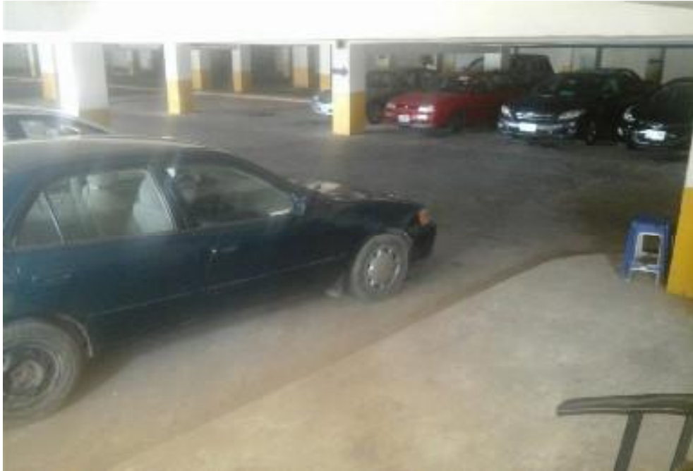
Plate 3.8: Basement car park, Heritage mall, Ibadan
