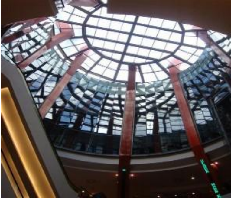
Plate 2.11: Daylighting from Skylights in Gordion AVM Ankara
