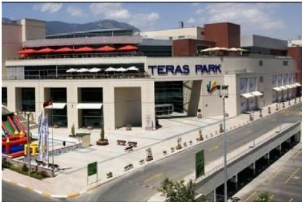
Plate 3.12: Exterior view of The Teras Park Shopping Mall, Denizli, Turkey
