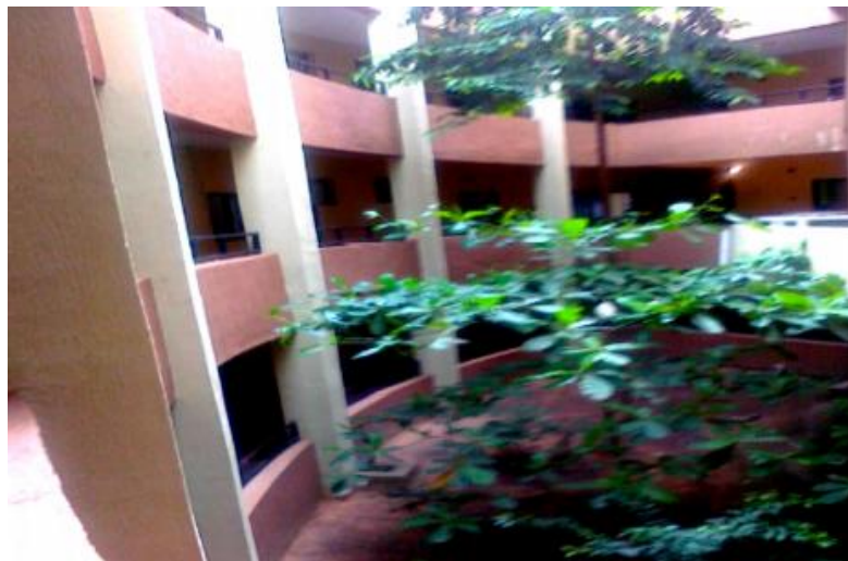
Plate 24: Courtyard view of LAUTECH Senate Building (Source –Author’s field work)
