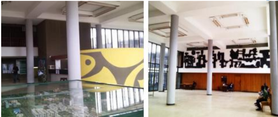
PLATE 10: Double volume space for reception, general waiting, and exhibition with 600mm diameter columns spaced @ 7m c/c (Source – Author’s field work)
