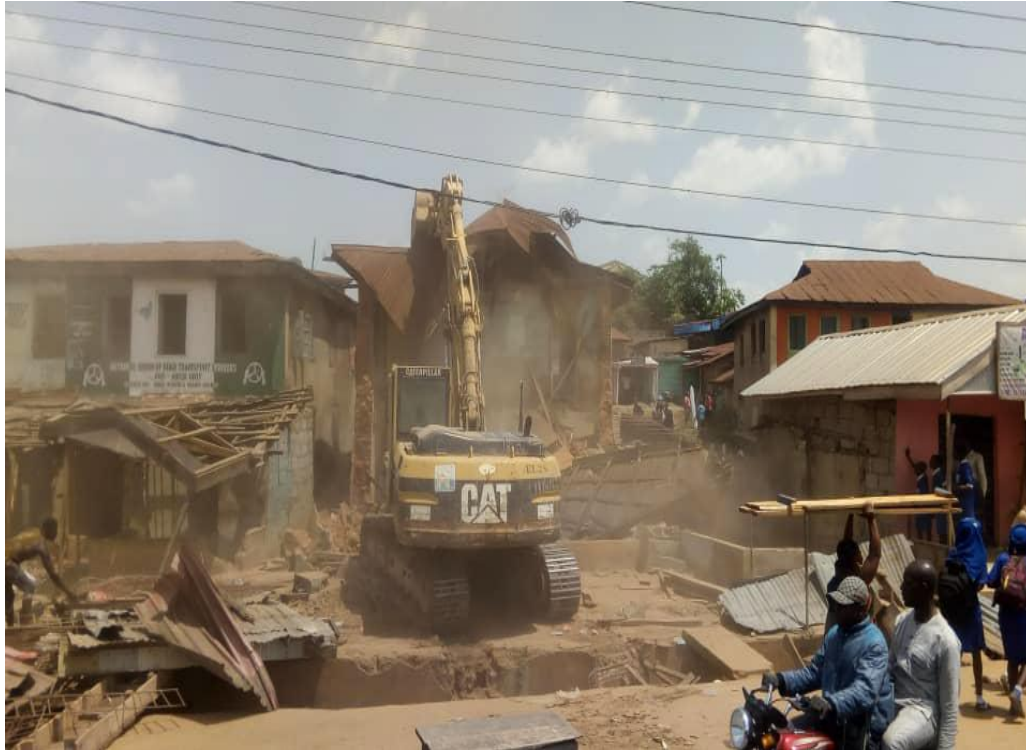
Plate 2.15: Demolition of an Urban Renewal Area Photo Credit: 7
