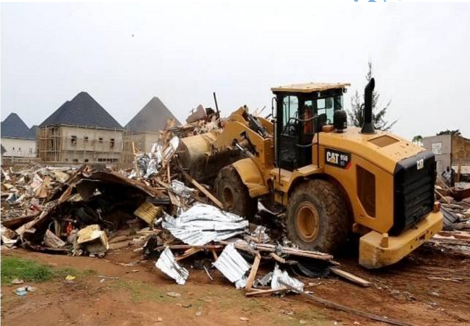
Plate 4.6: Demolition of Shops at DC Market, Phase IV, Kubwa, Abuja Photo Credit: The Authority Newspaper, 4 June 2023
