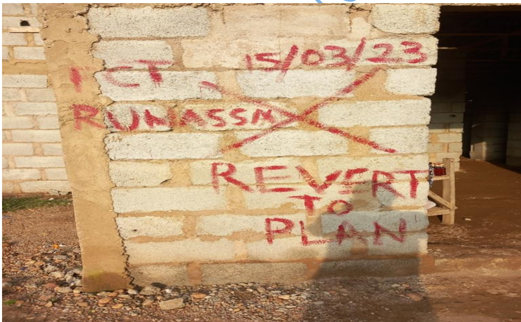
Plate 4.2: Ongoing Development “In Excess of Permit” at Jabi, Abuja Source: Author’s Fieldwork, (2023)
