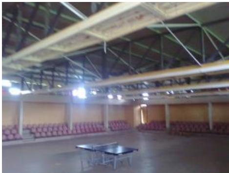
Figure 58: Interior view of the multipurpose court, O.A.U Sports Hall
