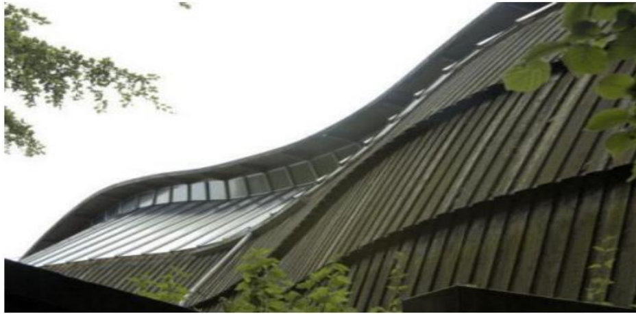
Figure 2.10: The Strategic Use of Clerestory Windows to Integrate Natural Lighting into a Museum Space
