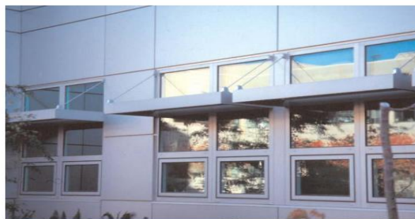
Figure 2.11: Light Shelf installation
