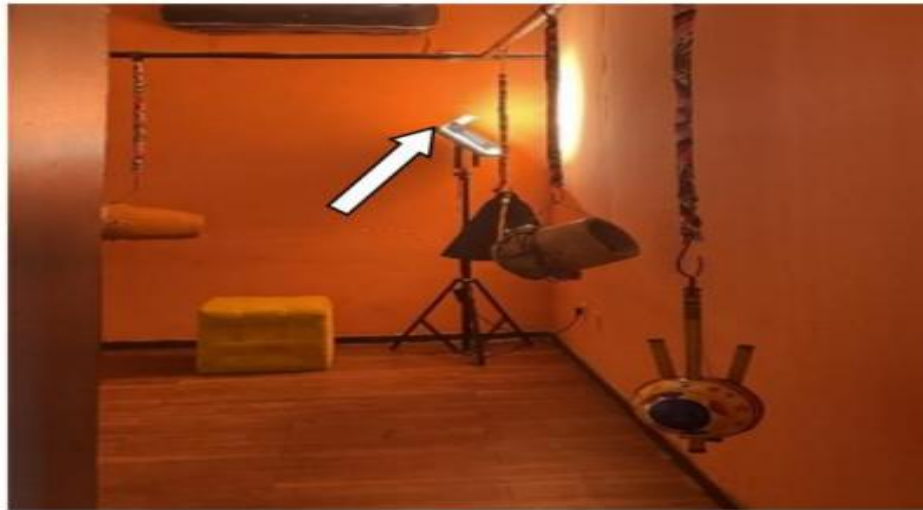
Plate 2.3: Up Lighting in a Display Area of the Discovery Museum, Wuse II, Abuja
