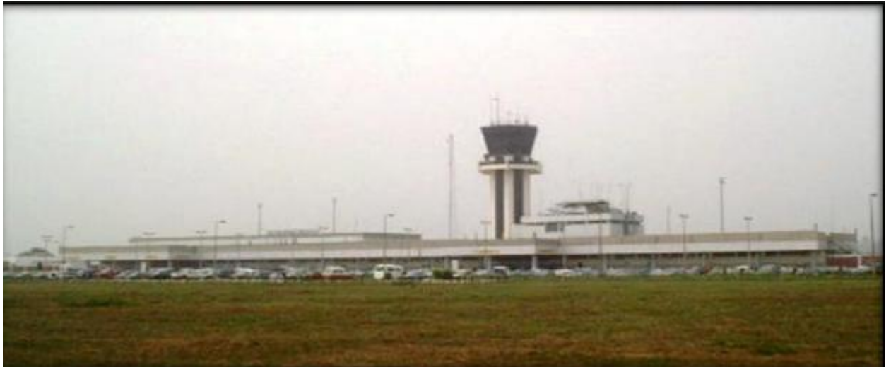
Figure 3.7b: PHC Airport Terminal building with the control tower Source: www.googleimages.com
