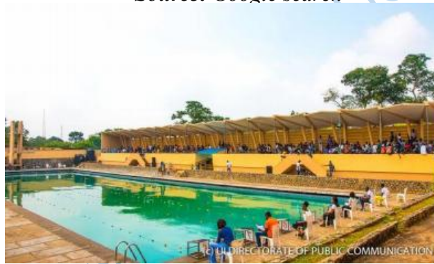
Plate 9: Interior view of the swimming pool for U.I Sport Hall
