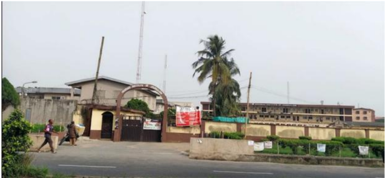
Plate 3.2: Nigerian Institute of Journalism, Ogba, Ikeja, Lagos (Wider View) Source: Authors field survey
