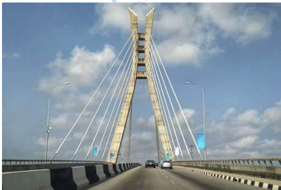
Plate 4.1: Lekki-Ikoyi Link Bridge Source: Authors Field work, 2024
