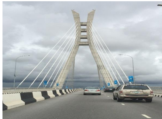
Plate 4.2: Lekki-Ikoyi Link Bridge Source: Authors Field work, 2024
