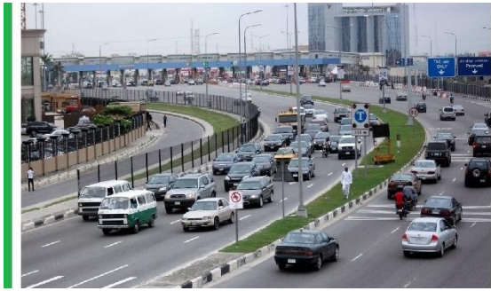
Plate 4.3: Lekki-Epe Expressway Source: Authors Field work, 2024
