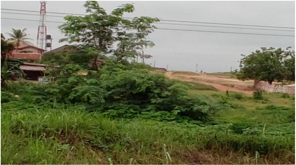
Figure 4.77. Buildings and Non-Compliance with Setbacks on Oil Pipeline in Ologuneru Area
