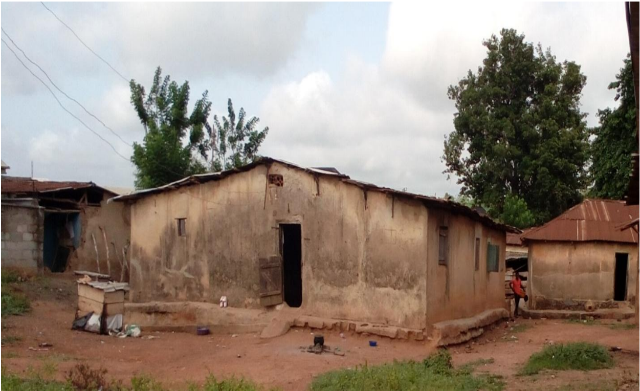
Figure 4.47 The Core Traditional Housing Type Still being Maintained by Original Land Owners in Alafara
