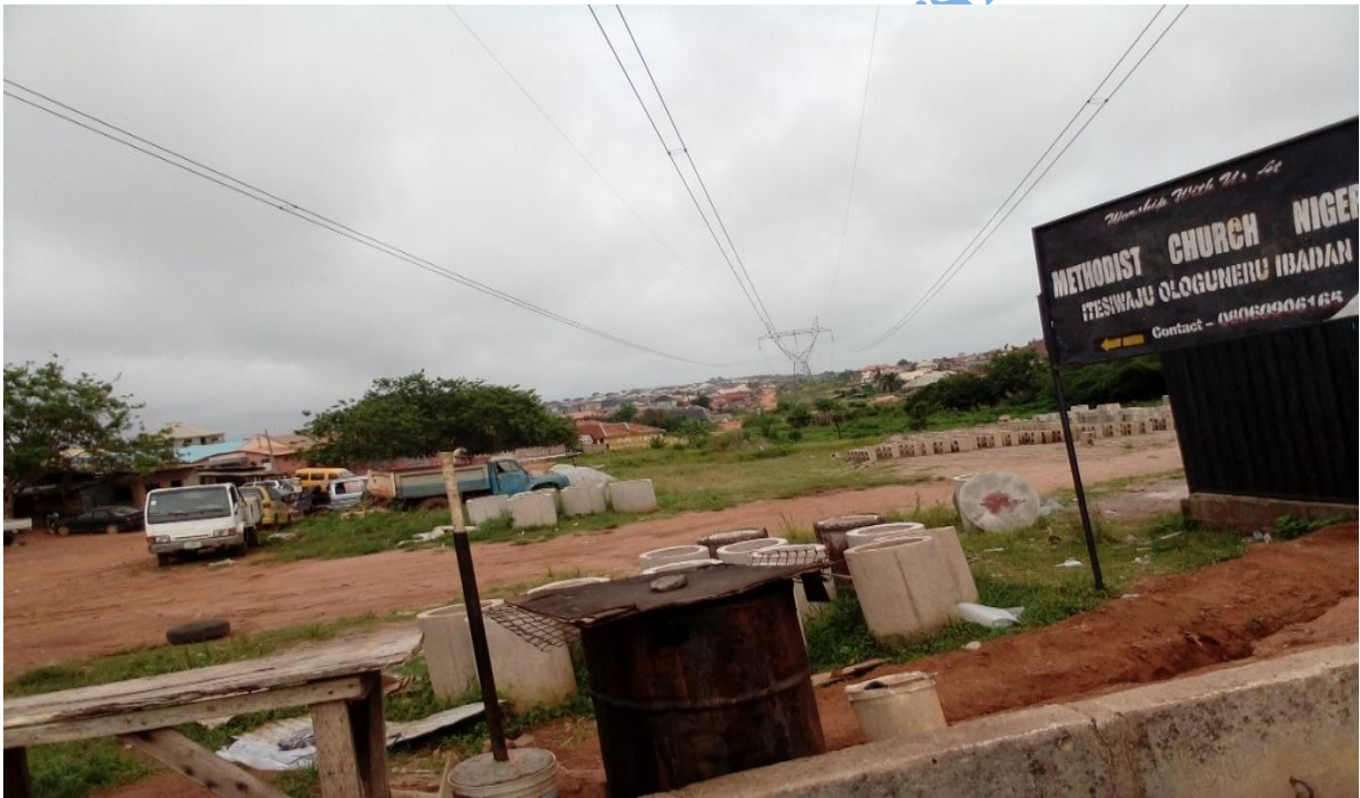
Figure 4.76. Buildings and Business Activities Under 33kva High Tension Wire
