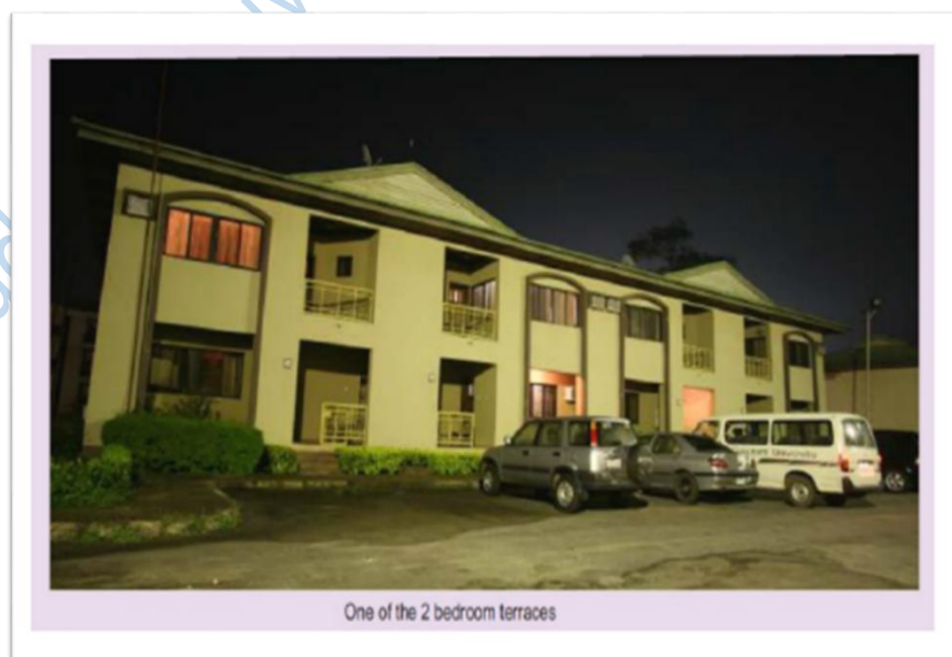
Plate 3.10: Illustrating University's Staff Quarters Building Showing a Typology
