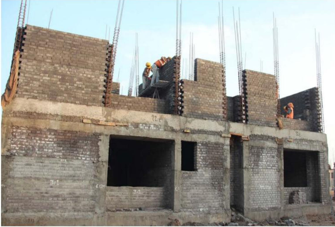
Housing during construction (Photograph by IIT Gandhinagar)
