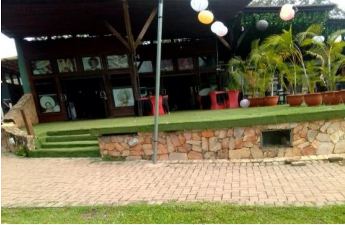
Figure 3.3 : View of the Musical stage Pavilion at Agodi Garden Entrance Gate
