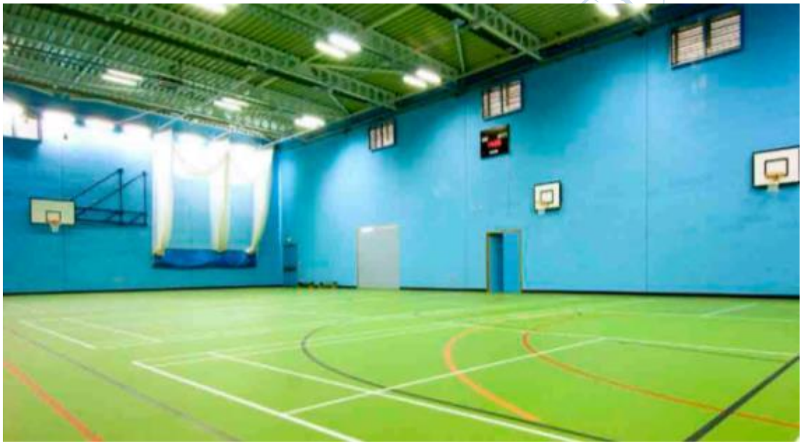
Figure 4.18: A combined elastic floor, wall of appropriate RV and compacts light between courts to Lighting System :
