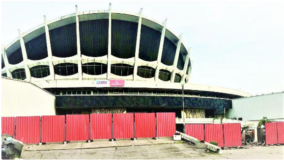
Figure 3.5: Side view of National Theater, Iganmu Lagos
