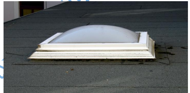
Figure 2.2: Skylights above lay lights
