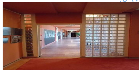
Figure 2.8: Open Floor designs and transparent Partitions
