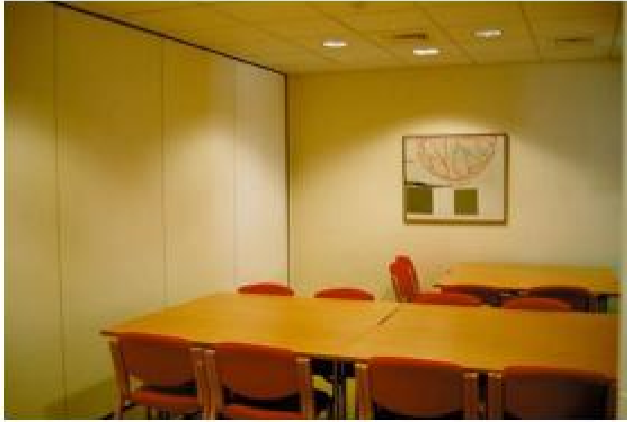
Figure 5: Stage 4 (Movable Acoustic Walls for Flexible Space)
