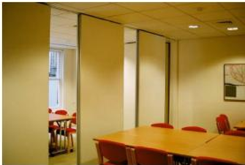
Figure 4: Stage 3 (Movable Acoustic Walls for Flexible Space)
