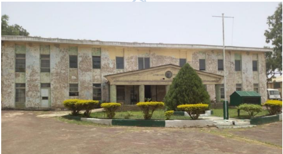
Figure 31: Figure 18: View showing the Administrative block. Source: Researcher's fieldwork (2022)
