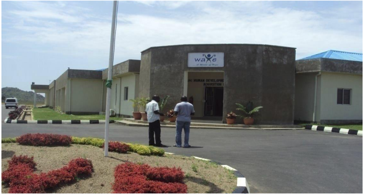
Figure 19: Approach View. Source: Researcher's fieldwork (2022)
