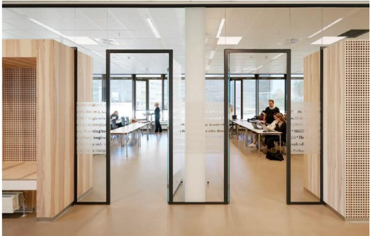
Figure 28: Interior view of the building showing non load-bearing demountable walls
