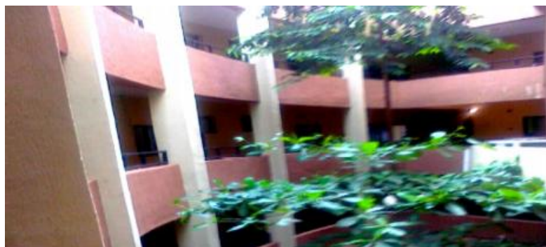
Plate 23: Rear view of LAUTECH Senate Building (Source –Author’s field work)
