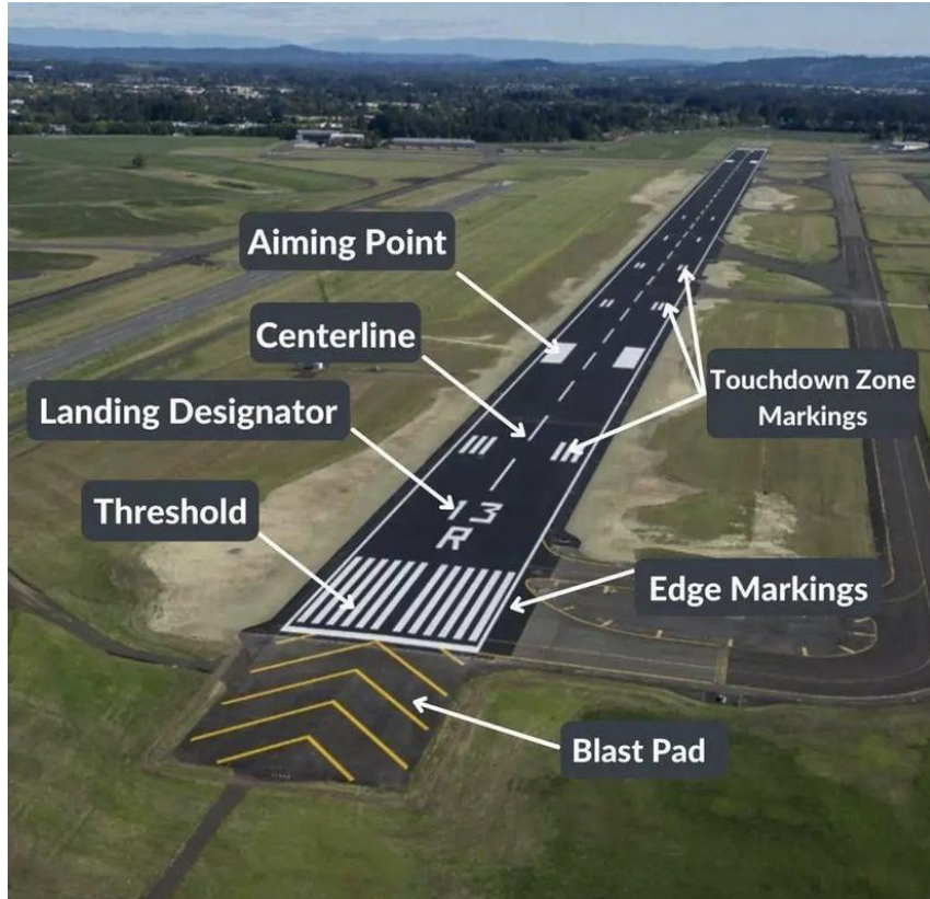
Plate 3. 13: Airport runway signage, and marking Source: www.reddit.com
