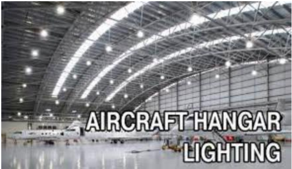
Plate 3. 16: Hangarage lighting arrangement Source: www.reddit.com
