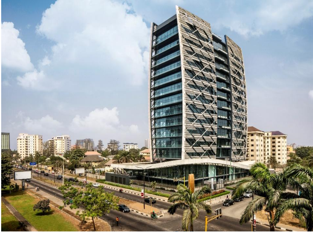
Figure 3.12: Exterior of Kings Tower Building
