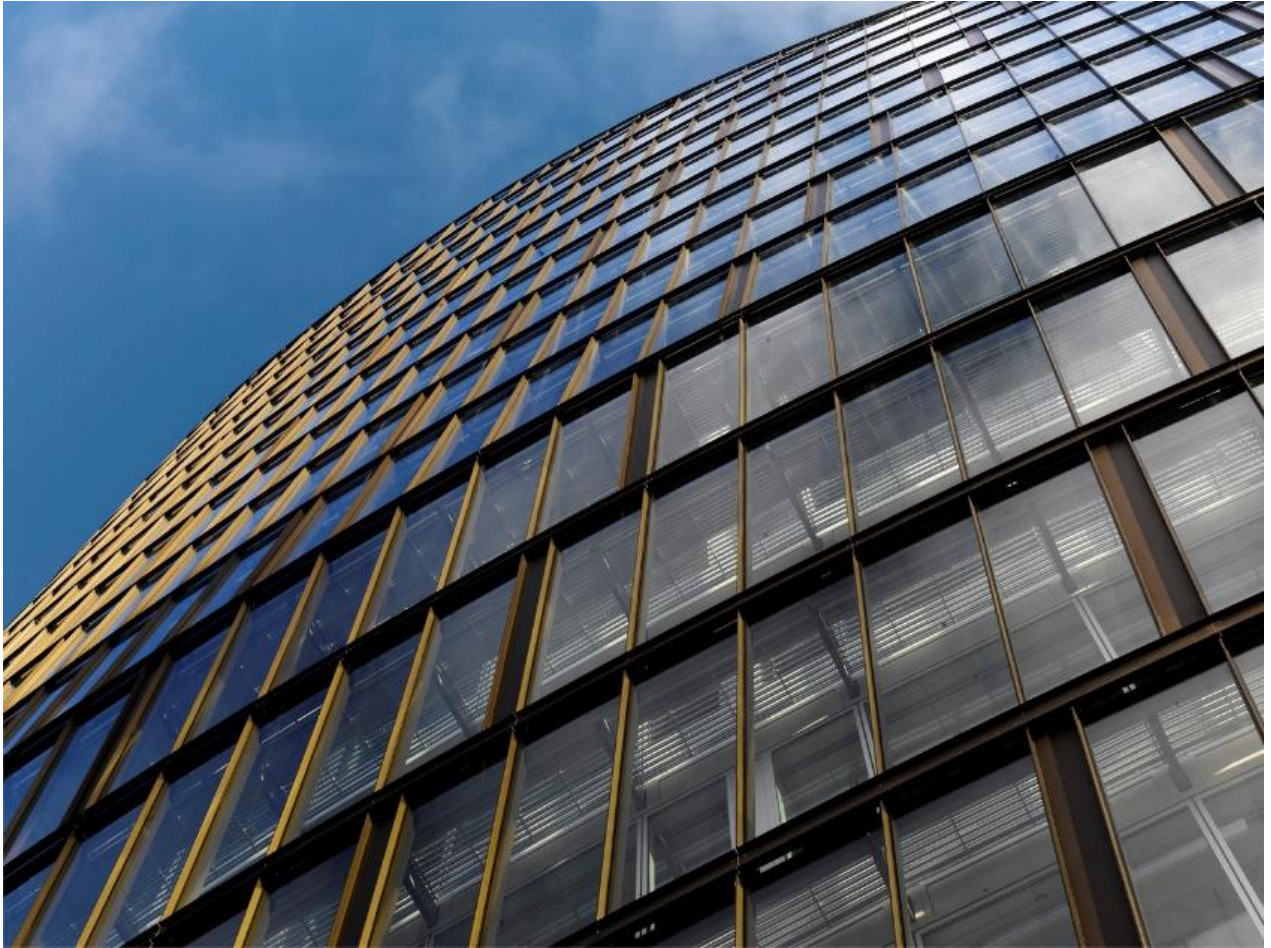
Figure 3.3: Exterior of Building Showing Façade of One Angel Square
