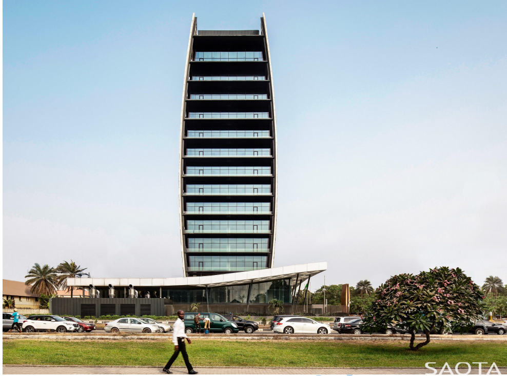
Figure 3.13: Exterior of Kings Tower Building
