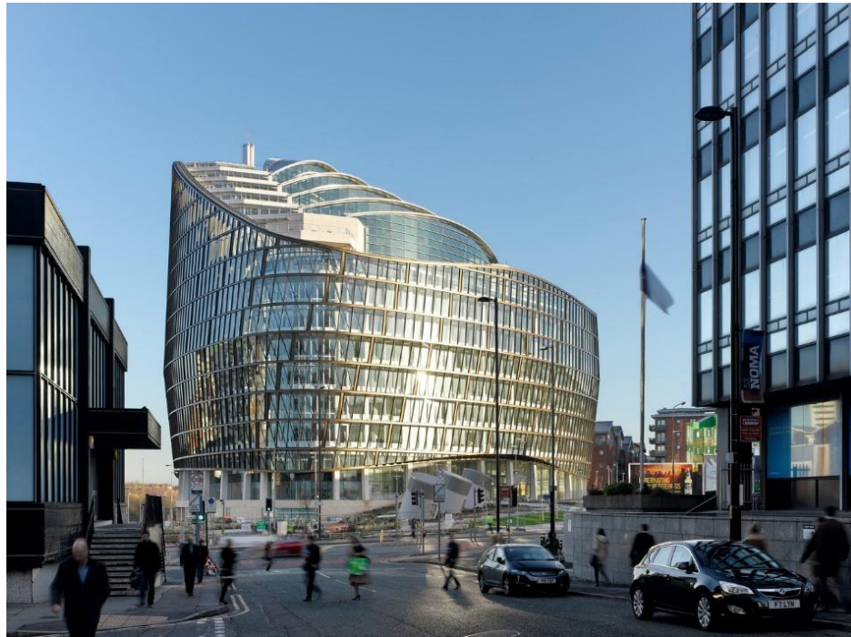
Figure 3.1: Exterior of One Angel Square Building
