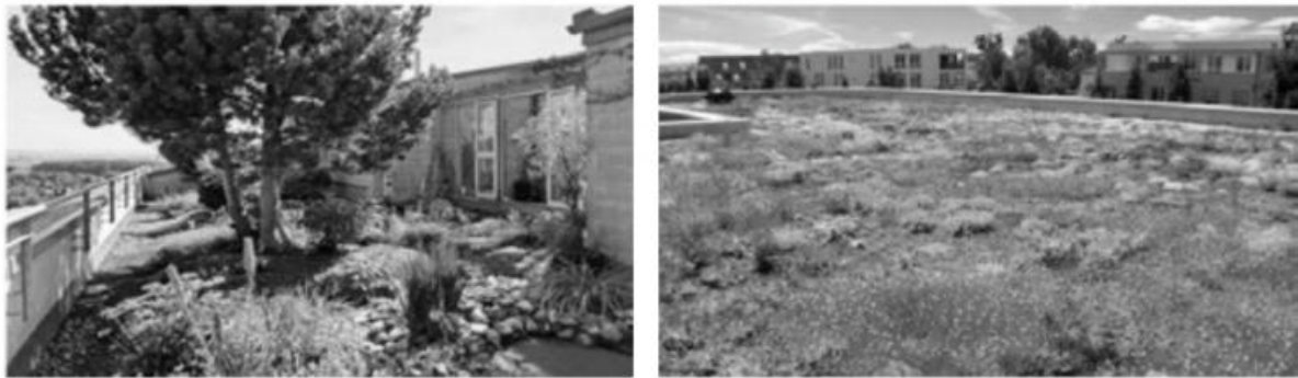
Plate 2.15. Intensive roof garden (left) and extensive roof plantings (right) ( Gülgün et al, 2015).
